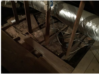
Approximate Average Depth of Insulation: Less than 4 Inches
