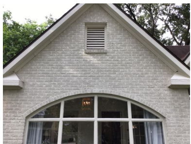
Type of Attic/Roof Ventillation: Gable vent, Turbine vent
