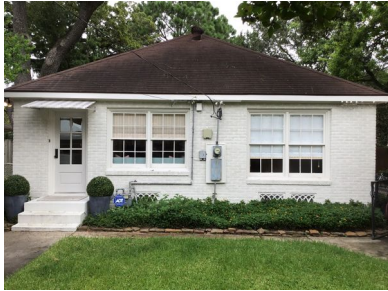
General Photos of Roof Covering:
