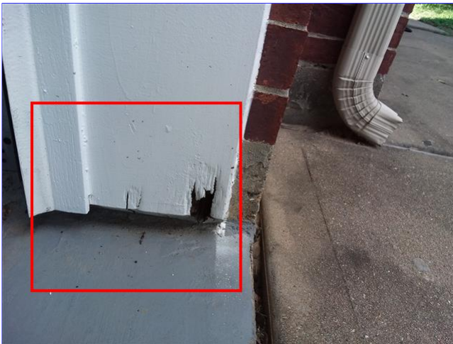
F. Item 3(Picture) Wood rot was discovered at the base of both garage doors frames.
