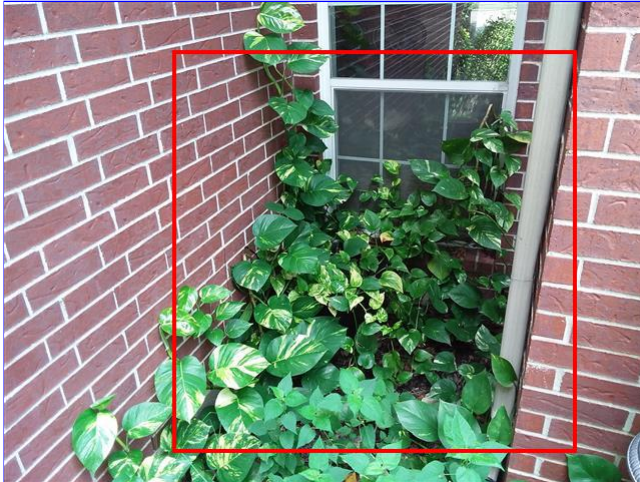
B. Item 1(Picture) Vegetation should not be on the structure.
