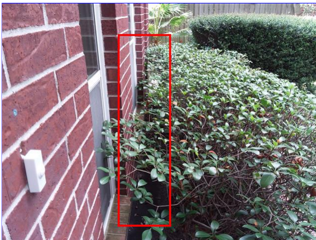
B. Item 2(Picture) Vegetation at the front of the home is too close to the structure.
