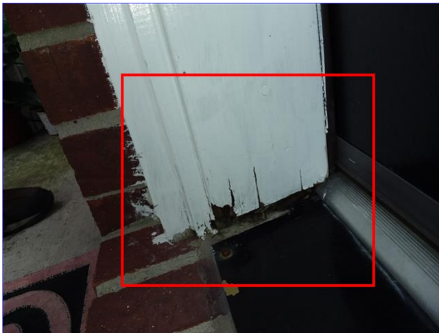
F. Item 5(Picture) Wood rot is discovered at the front door frame base.
