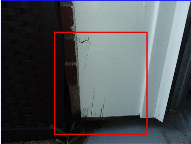
F. Item 2(Picture) Wood rot was discovered at the base of both garage doors frames.
