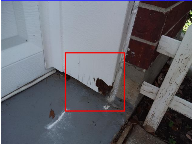
F. Item 4(Picture) Wood rot was discovered at the base of both garage doors frames.
