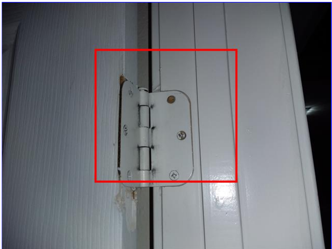
F. Item 9(Picture) Hinge screw is missing from second floor left front bedroom.
