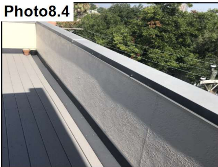
Metal caps are present at terrace.
