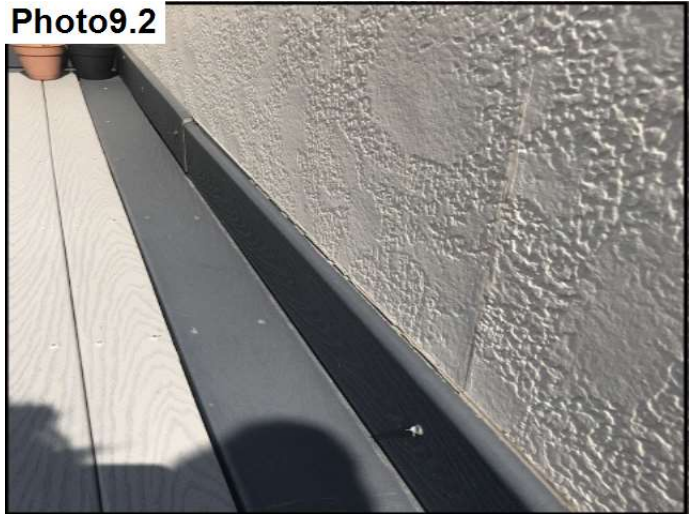
Seal balcony floor terminations as needed.
