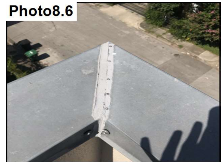
Reseal metal cap joints and transitions as needed.
