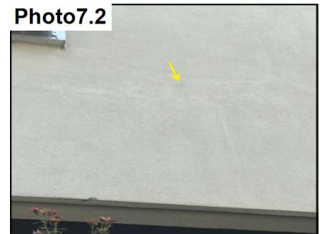
Photo7.2 Hairline cracks are present.
