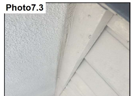
Photo7.3 Reseal siding transitions as needed.
