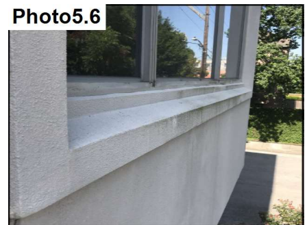
Apply elastomeric coating on top of semi-flat wall.
