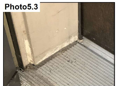
Reseal door miters as needed.
