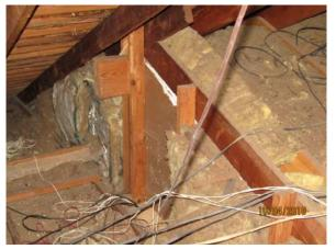
• Missing vertical bracings, under sized purlins, missing purlins, and sagging structure were viewed in the attic area. Strengthening the roof structure would improve structural integrity and resist future movement. While this improvement is not considered priority, it can often be accomplished without a great deal of difficulty.
