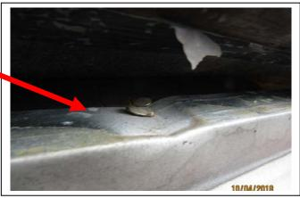
• The water heater and furnace vent pipe storm collars are missing and water is entering the attic during rainy conditions. Sealant repairs are needed.
