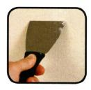
5 Small cracks in sheetrock are a natural occurrence when a home's moisture stabilizes. Homeowner applied caulk or spackle will correct these small cracks.
