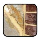
Hairline cracks in the mortar of new construction are expected and are not considered a defect.
