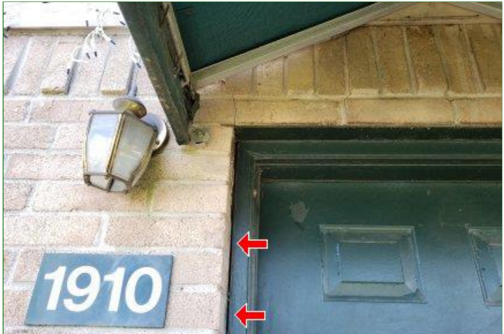
2.1 Item 1(Picture) seal around door frame
