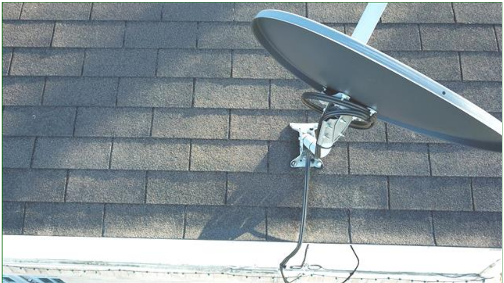
1.0 Item 8(Picture) Roof covering materials
