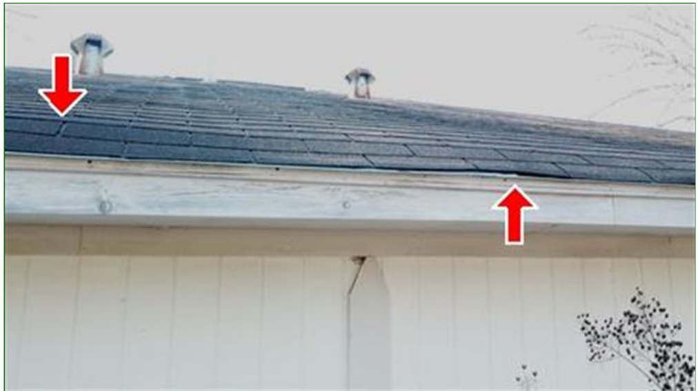
2.5 Item 10(Picture) Roof decking at rear of building
