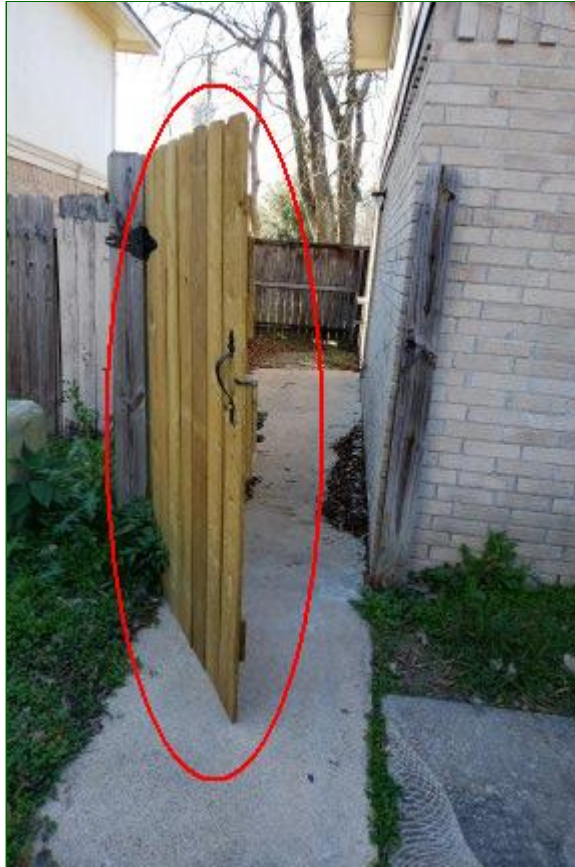
2.4 Item 3(Picture) Gate must be lifted to open and close and is in need of repair.
