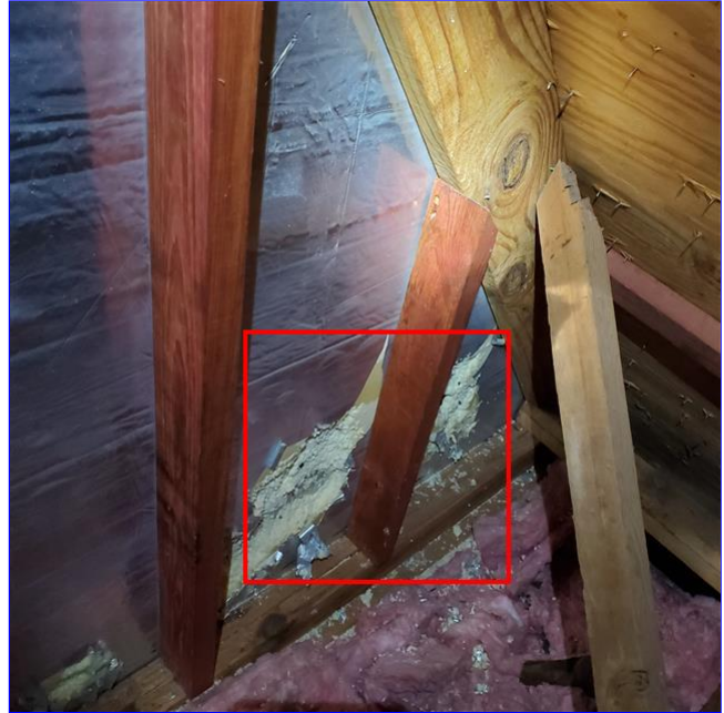
L. Item 2(Picture) Possible evidence of critters was noted in the attic. No critters were noted in attic at time of inspection but should be evaluated further.
