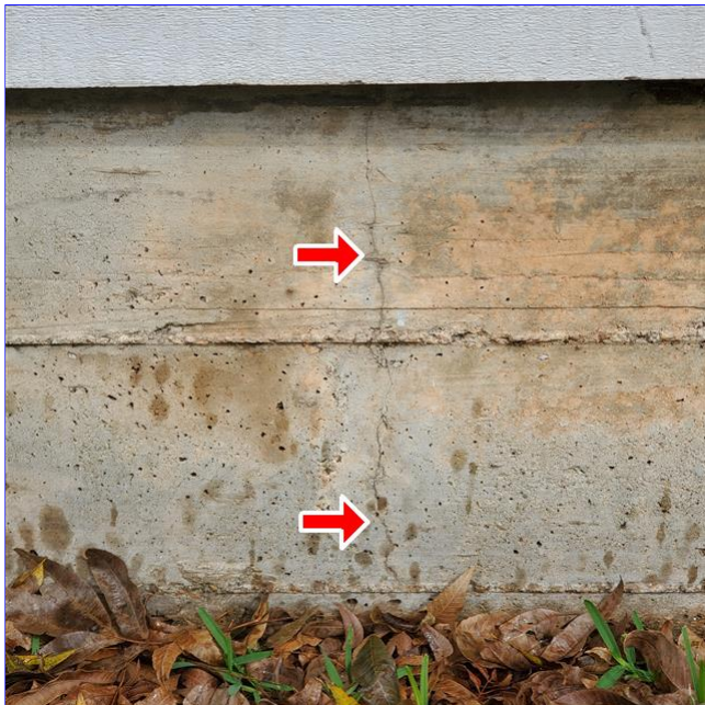
A. Item 3(Picture) Hairline crack in the foundation at the back of the home by the master bathroom.
