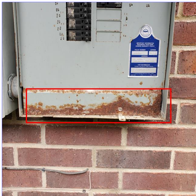
A. Item 1(Picture) The dead front cover on the electrical panel is Rusted and should be repaired/ replaced to help prevent further damage.
