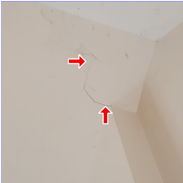
F. Item 3(Picture) Fairly large crack in the living room ceiling. This crack may not be cosmetic and should be evaluated further.
