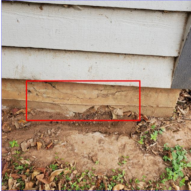
A. Item 1(Picture) Damage foundation at the back of the garage needs repair.
