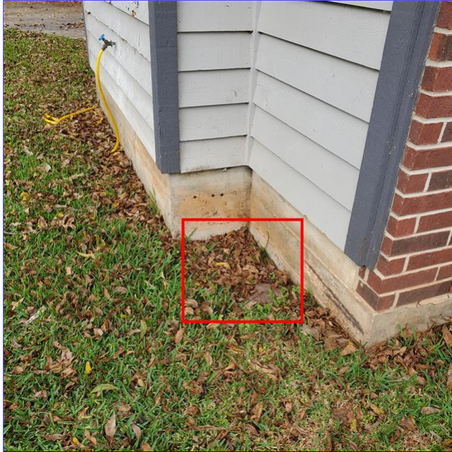
B. Item 5(Picture) area for potential ponding water at the back of the home by the master bathroom.
