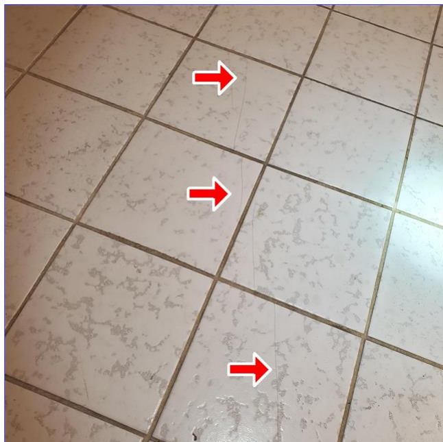
F. Item 5(Picture) Hairline cracks noted and tile at the front entrance. I'm sure if this is cosmetic or structural but does not appear to be severe at the moment but should be evaluated and repaired, if needed.
