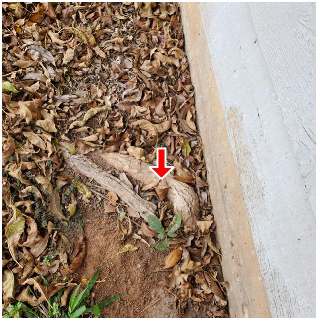
L. Item 3(Picture) Tree root growing under the foundation of the garage at the left side of the garage.
