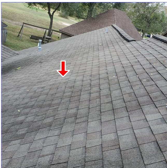
D. Item 7(Picture) Slight hump in roof structure on the back facet approximately above the living room. This is approximately where the fairly large crack in the ceiling is and needs further evaluation.
