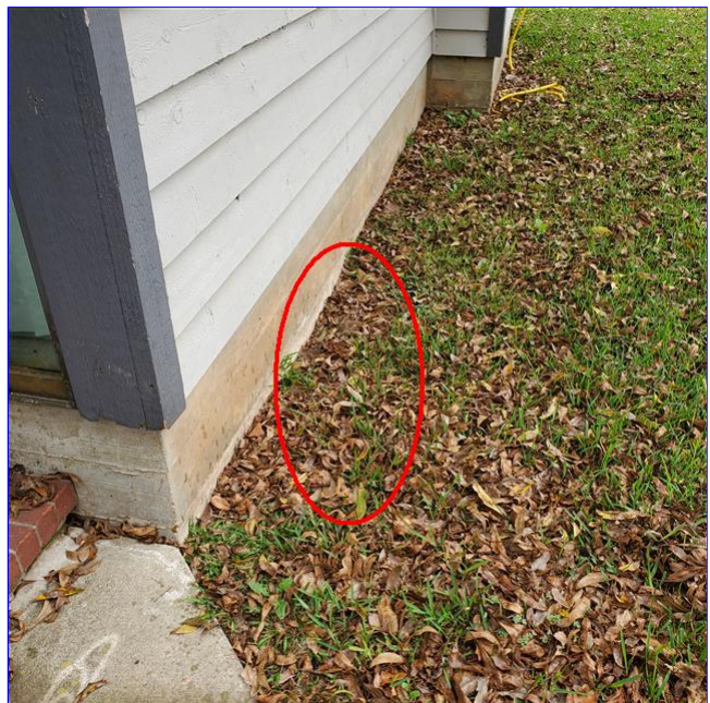
B. Item 4(Picture) Area for potential ponding water at the back of the home by the master bedroom.
