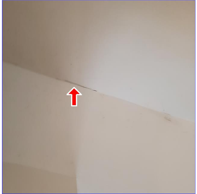
F. Item 2(Picture) Tape peeling from the ceiling in the living room appears cosmetic but should be sealed and monitored.
