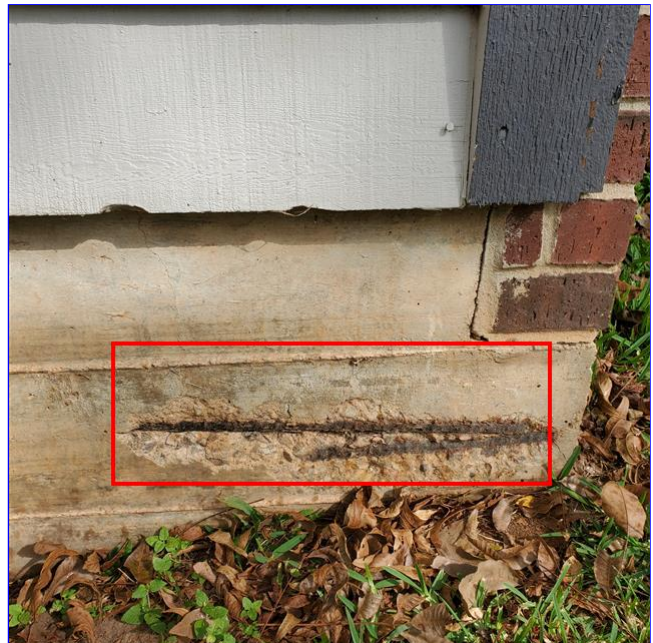
A. Item 4(Picture) exposed rebar in foundation at the back left corner of the home needs repair to help prevent further damage.
