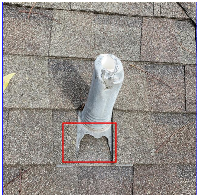
C. Item 4(Picture) Damaged vent pipe flashing on vent pipe approximately above the master bathroom.
