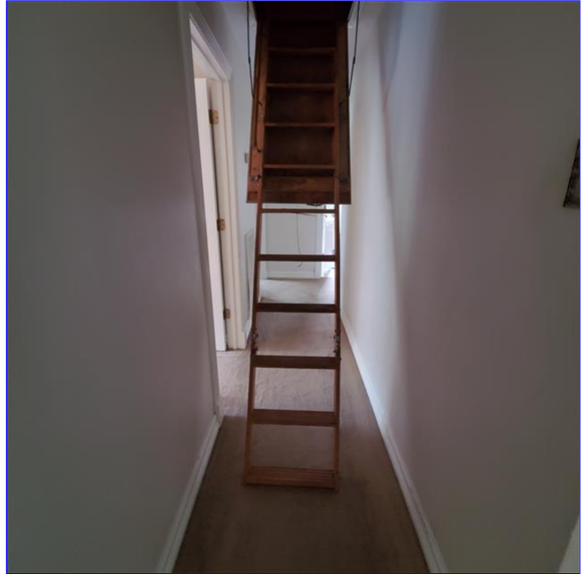
D. Item 2(Picture) The attic ladder is aged in flimsy and should be replaced for safe entry into the attic.
