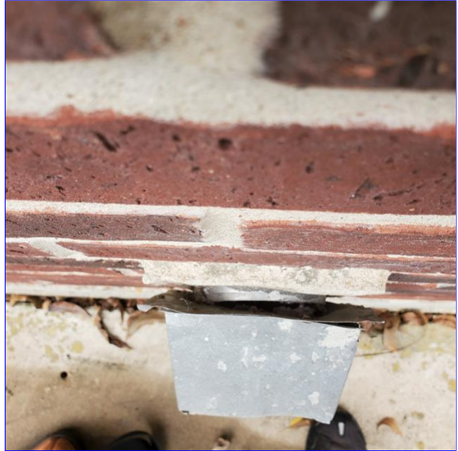
H. Item 2(Picture) The exterior of the dryer exhaust vent is loose and needs to be secured.
