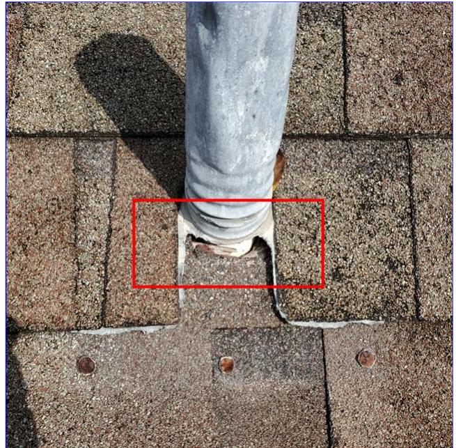
C. Item 2(Picture) Damaged pipe flashing approximately above the kitchen needs repair.
