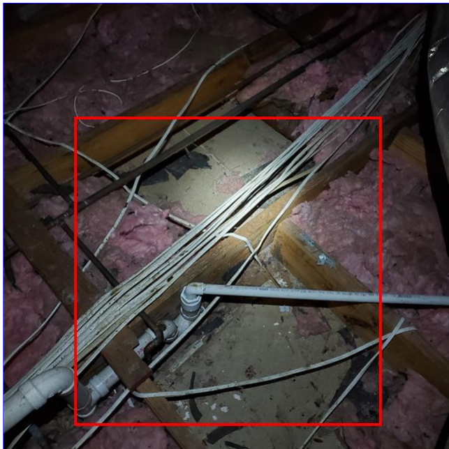
D. Item 3(Picture) Voids in attic insulation approximately above the hallway bathroom.
