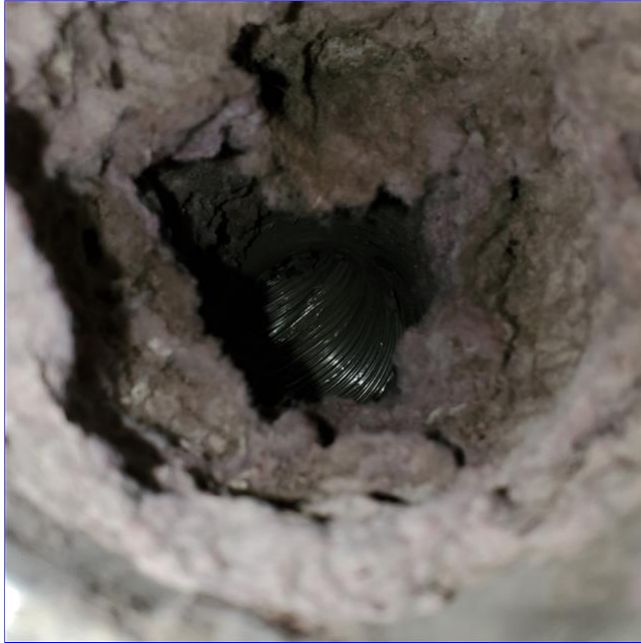
H. Item 1(Picture) The dryer exhaust is full of debris and needs to be cleaned to help prevent possible fire hazard.
