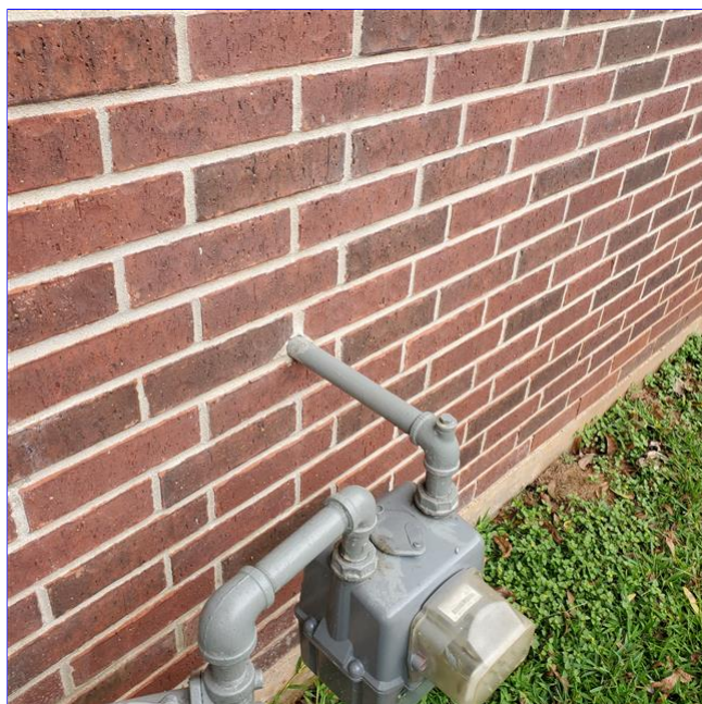
A. Item 3(Picture) Above-ground gas piping is not bonded to the grounding electrode system.
