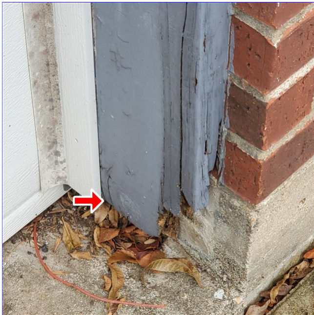
E. Item 7(Picture) Rotting trim was noted on both sides of the garage door on the left and needs repair.
