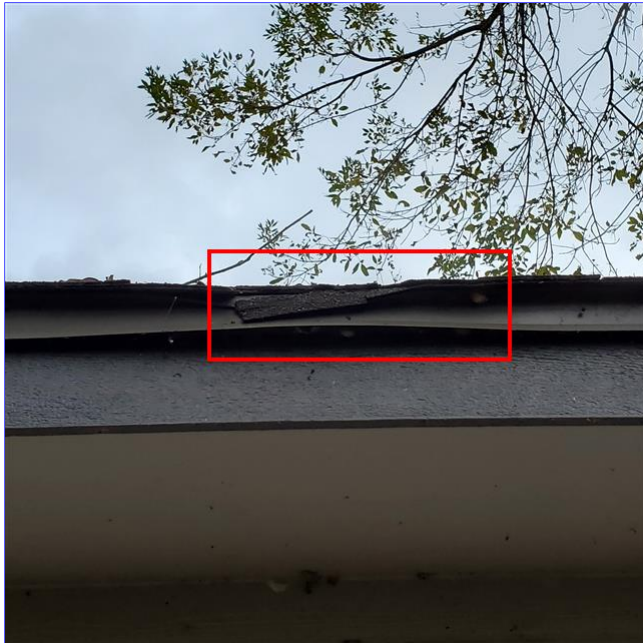
C. Item 1(Picture) Damaged shingle and bent drip edge at the back facet of the garage.
