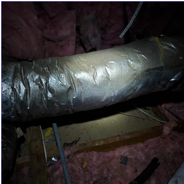
D. Item 5(Picture) Void in insulation approximately above the hallway.
