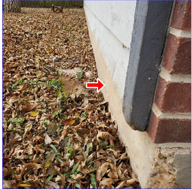
A. Item 2(Picture) Bowed foundation wall at the left side of the garage near the front entrance door of the garage. This needs further evaluation by professional contractor and repair, as needed
