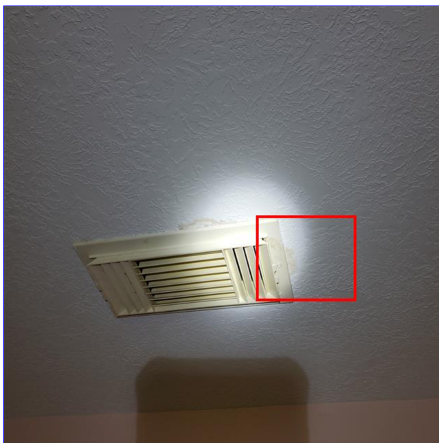
F. Item 8(Picture) Stain on ceiling around vent register in the bedroom to the left at the end of the hallway.
