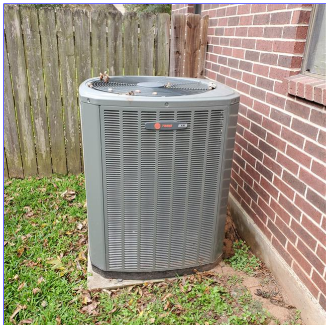
B. Item 4(Picture) General view of AC condenser. This unit was manufactured in 2015, typical life expectancy is 15 to 20 years.
