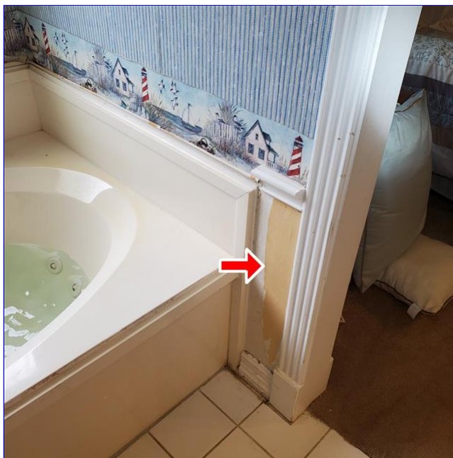
E. Item 2(Picture) Cosmetic damage to wall in the master bathroom by the HydroMassage tub. Evaluate and repair, as needed. Also recommend caulking between the wall and the HydroMassage tub to help prevent water from entering this area and causing damage to property
