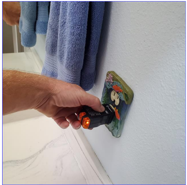
B. Item 4(Picture) Electrical receptacles in the hallway bathroom or not GFCI protected and need to be replaced for safety.
