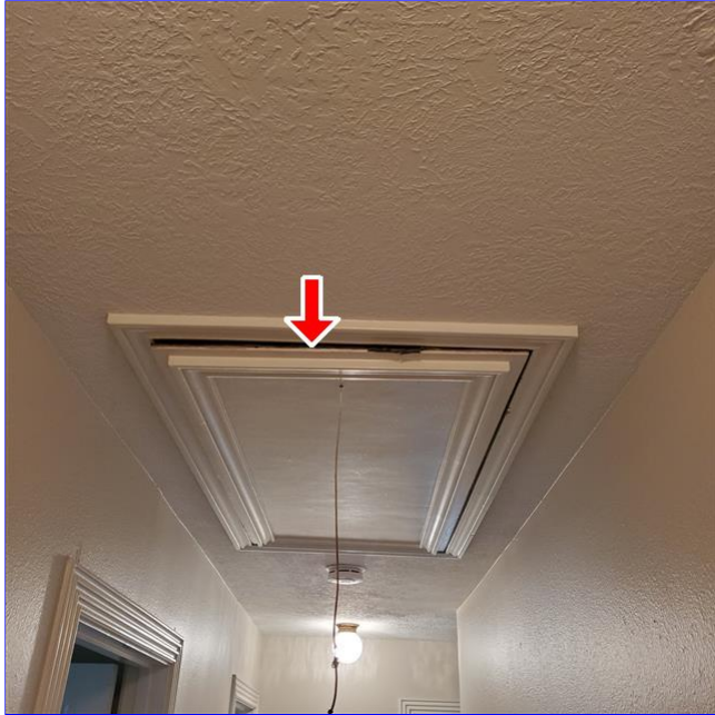
D. Item 1(Picture) Gap in the attic access needs to be sealed to help prevent loss of conditioned air.
