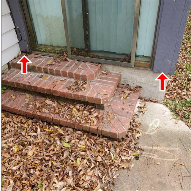
E. Item 5(Picture) Rotting trim by the master bedroom sliding glass door needs repair.
