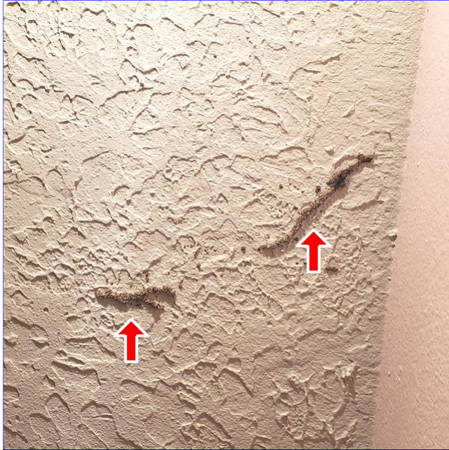
L. Item 1(Picture) Evidence of possible wood destroying insects was noted in the closet of the bedroom to the left at the end of the hallway.
