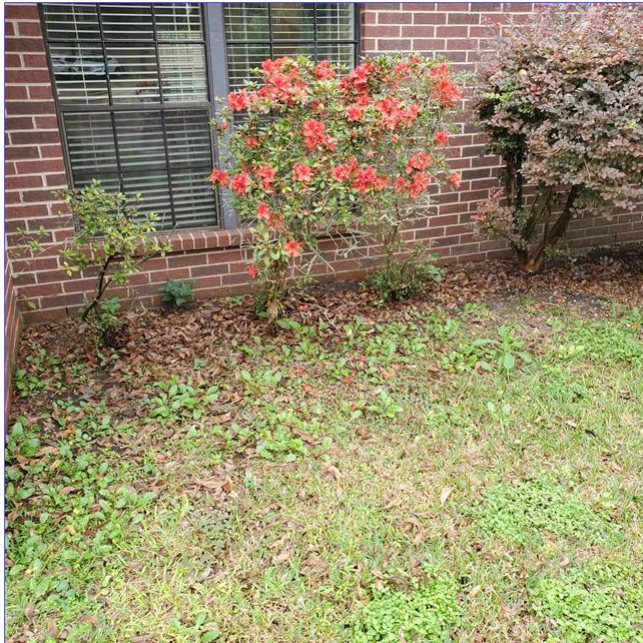
B. Item 1(Picture) The soil at the front of the home is within 4in of brick wall coverings and needs to be lowered.
