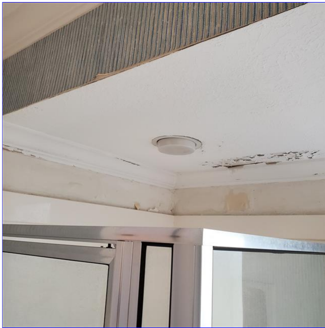
B. Item 3(Picture) The light above the master bathroom shower was not working at time of inspection and needs further evaluation.
