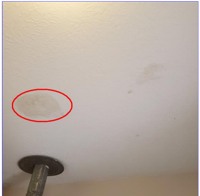
F. Item 4(Picture) Water stains noted on the ceiling in the laundry room. This did not appear wet at time of inspection but should be monitored.
