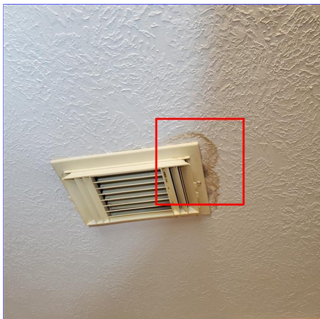
F. Item 7(Picture) Water stain around vent register in the hallway bedroom on the right at the end of the hallway is possibly due to condensate event, however, this area was not wet at time of inspection and should be further evaluated and monitored, at minimum.
