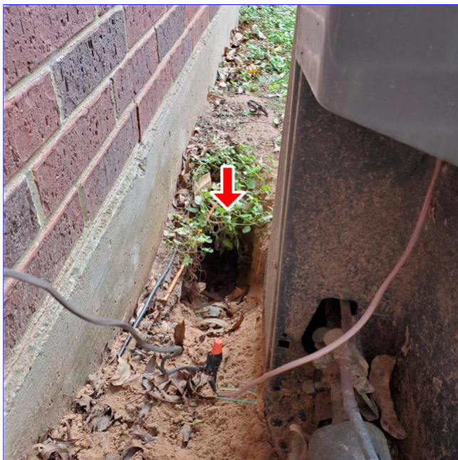
B. Item 3(Picture) Possible critter hole going under the foundation at the left side of the home by the AC condenser. This needs remedy to help prevent moisture from entering under the foundation and causing damage.
