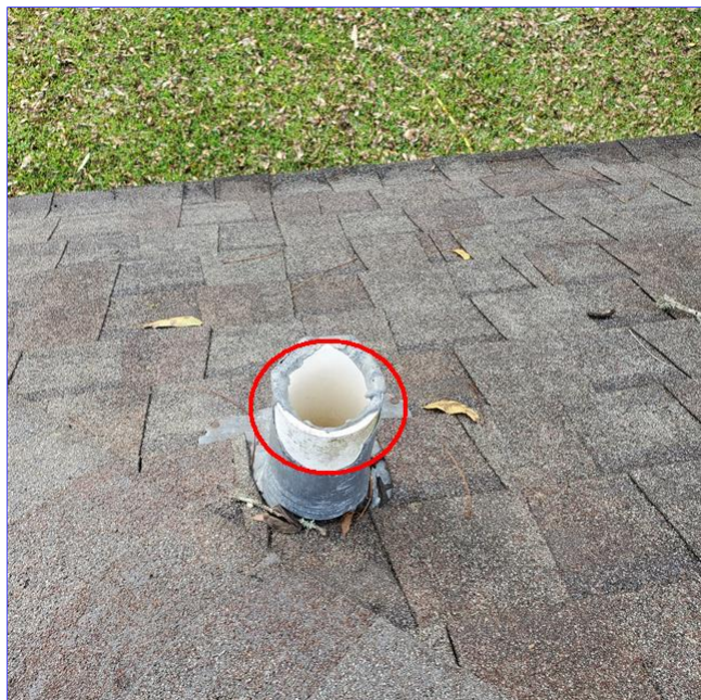
C. Item 5(Picture) Damaged vent pipe flashing on vent pipe approximately above the master bathroom toilet.
