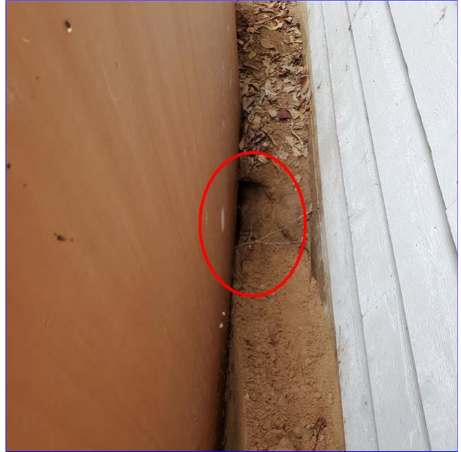
B. Item 6(Picture) Possible critter hole going under the foundation at the right side of the garage.
