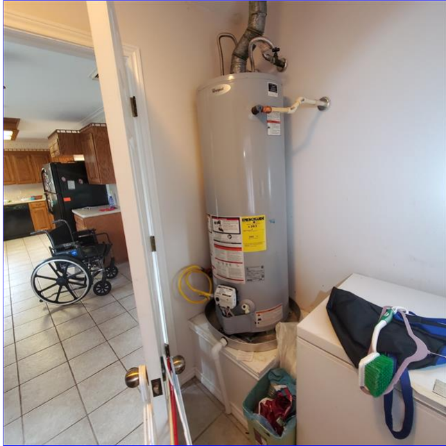
C. Item 1(Picture) General view of Whirlpool 40 gallon gas water heater. this unit was manufactured in 2015, typical life expectancy is 8 to 12 years.
