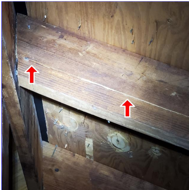
D. Item 6(Picture) Split rafter noted in the attic at the vaulted ceiling in the living room.
