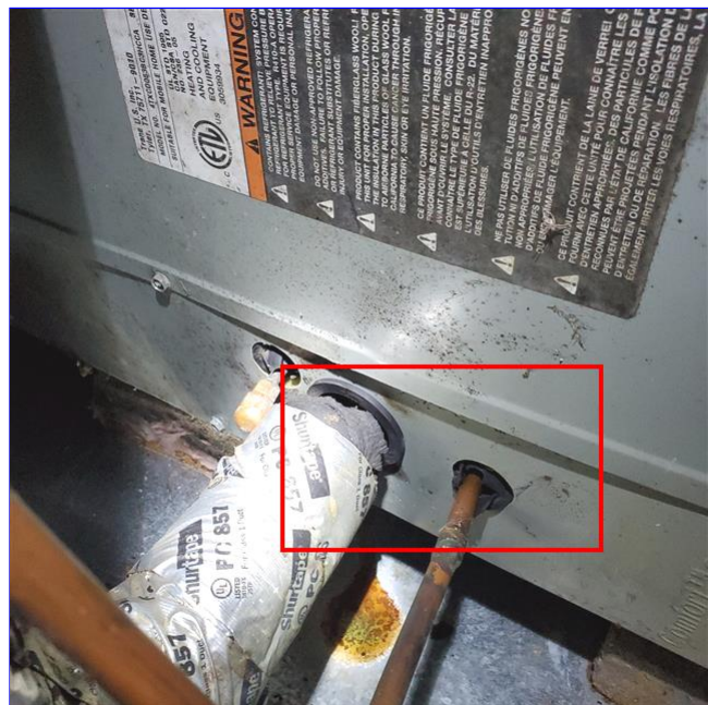
B. Item 3(Picture) There are gaps around the coolant lines at the evaporator coil, in the attic, that need to be sealed to help prevent condensation in this area.
