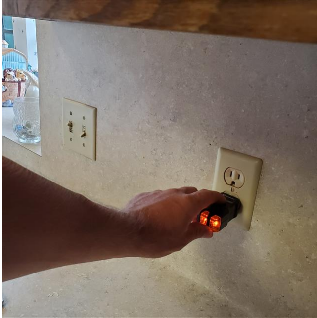
B. Item 1(Picture) Electrical receptacles above kitchen counter tops are not GFCI protected. This may not have been required when the home was built and his grandfather again what is the current requirement for safety.
