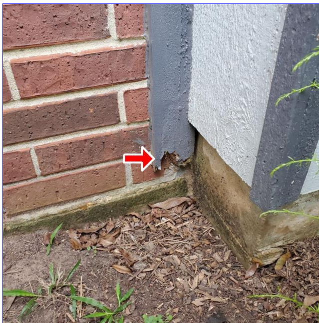
E. Item 4(Picture) Rotting trim at the front of the home, by the middle hallway bedroom window needs repair.
