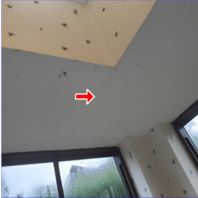
F. Item 1(Picture) Hairline crack in the ceiling above the kitchen sink appears cosmetic but should be sealed and monitored for growth and a structural engineer contacted if growth occurs.
