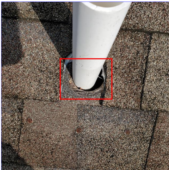
C. Item 3(Picture) Missing pipe flashing around plumbing vent pipe above the laundry room.
