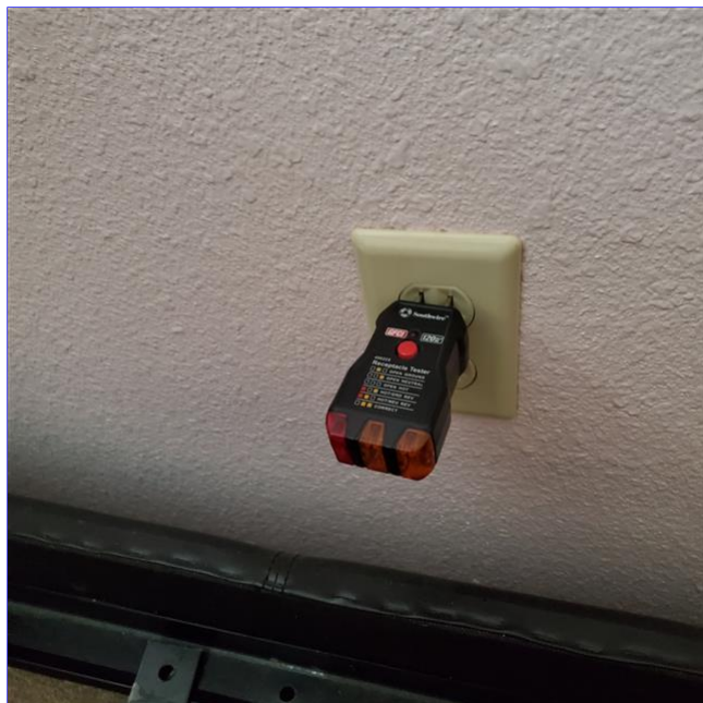
B. Item 5(Picture) Electrical tester could not be inserted in the top portion of the receptacle on the South Wall in the bedroom to the left at the end of the hallway. Unsure of cause but recommend further evaluation and repair.
