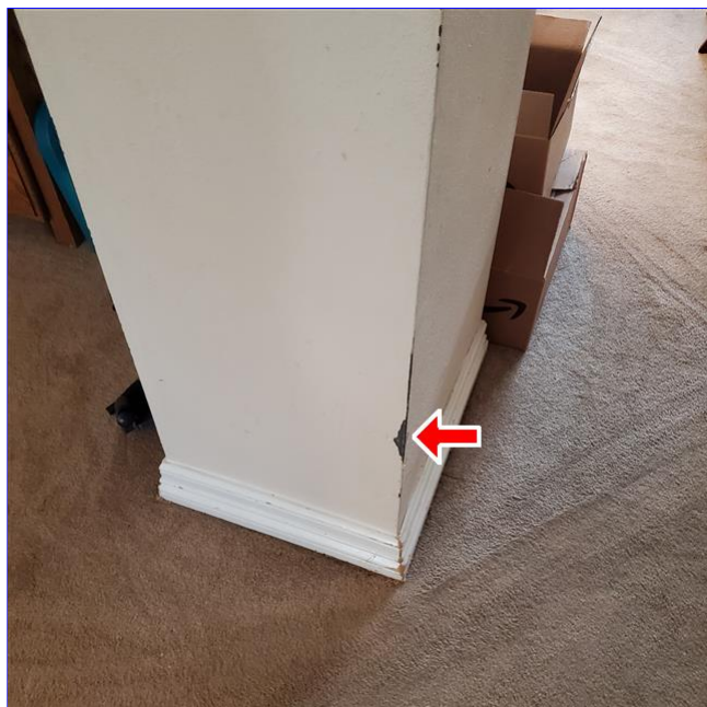
E. Item 1(Picture) Cosmetic damage to wall in the living room. Evaluate and repair as needed
