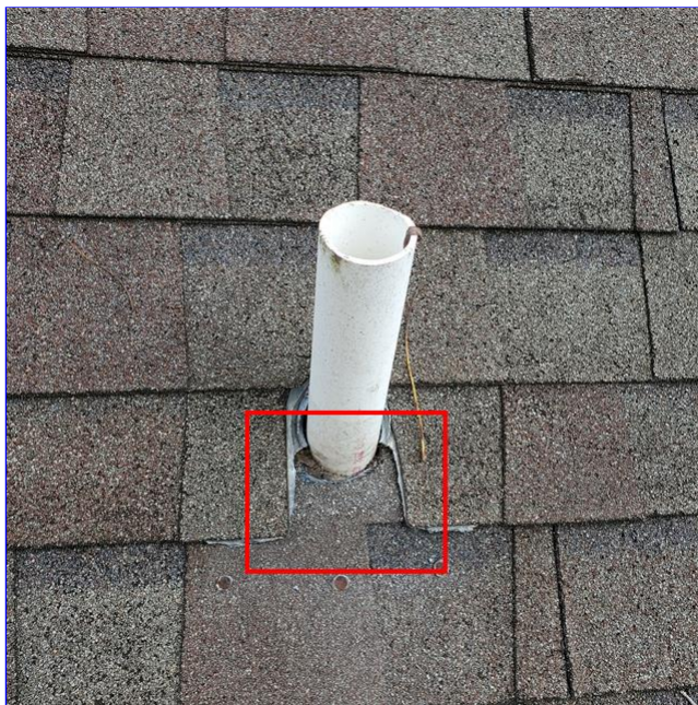
C. Item 6(Picture) Missing vent pipe flashing on vent pipe approximately above the hallway bathroom.
