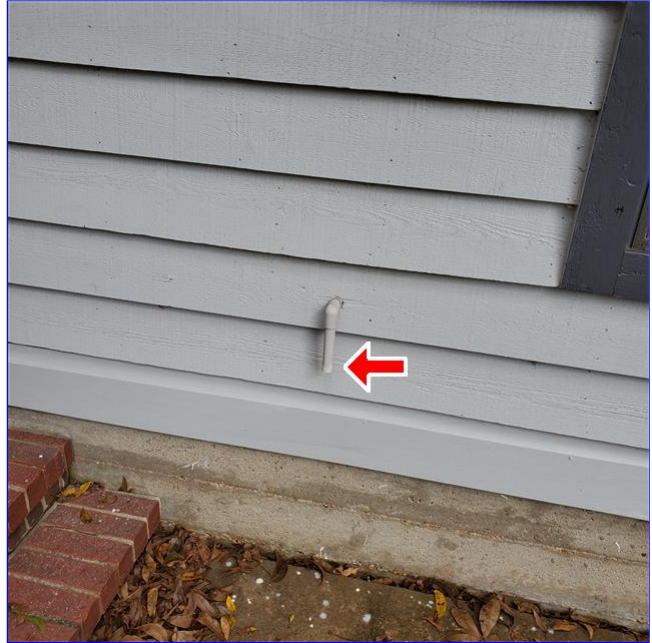
C. Item 2(Picture) TPR drain extension piping, at the back of the home, needs to be extended to within 6 to 24 in of the ground for safety.
