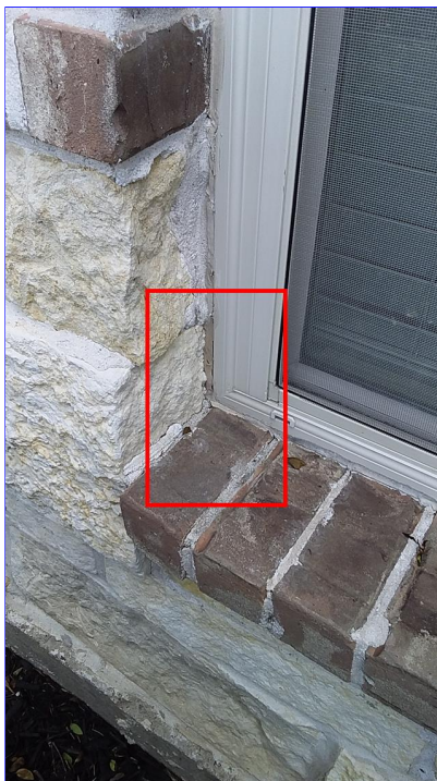
H. Item 2(Picture) multiple windows exterior
