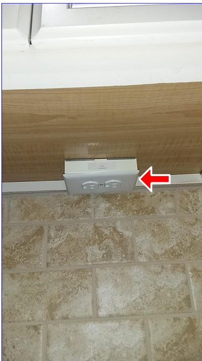
B. Item 5(Picture) kitchen outlets
