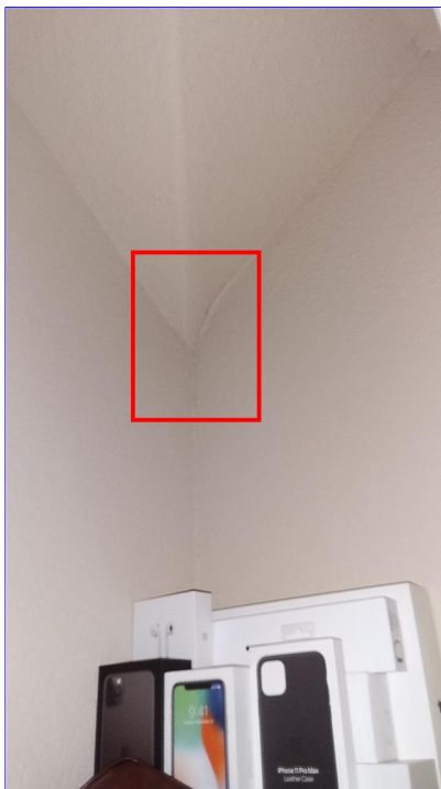
F. Item 4(Picture) left front bedroom closet
