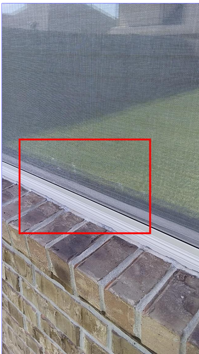
H. Item 6(Picture) rear
