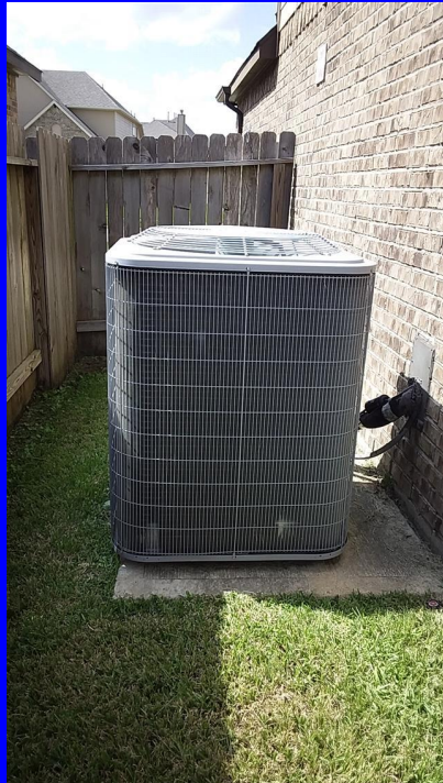
ac unit exterior right
