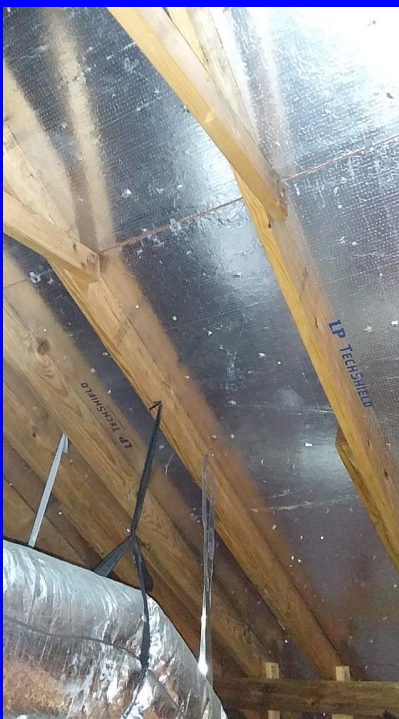
stick built roof structure with radiant barrier
