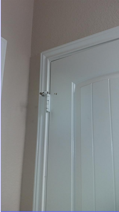
G. Item 1(Picture) left bath upstairs
