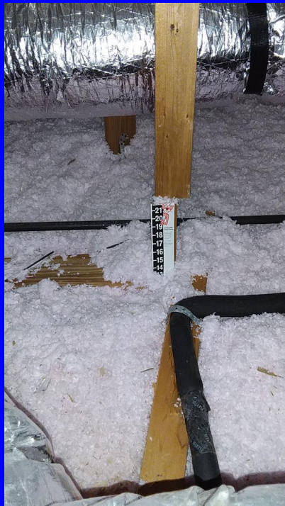
blown insulation 12 inches
