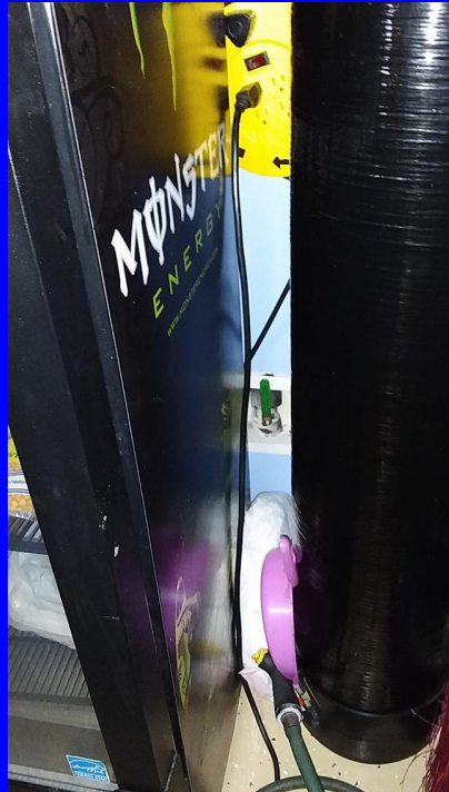
water shut off garage right
