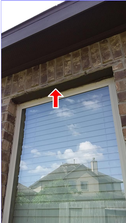
H. Item 5(Picture) rear
