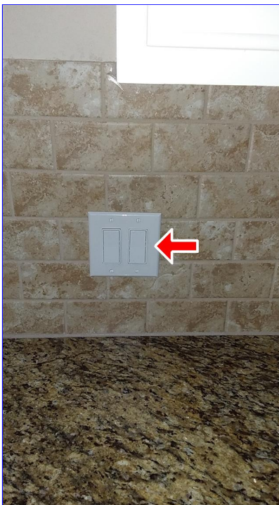
B. Item 8(Picture) right of kitchen sink
