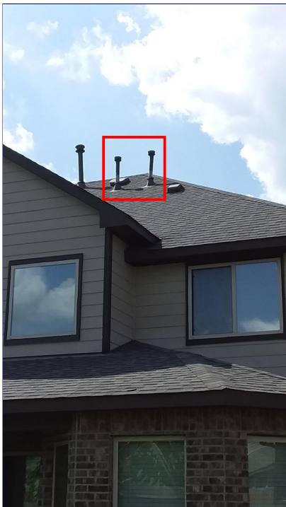
C. Item 6(Picture) rear
