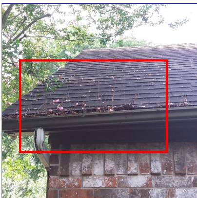
B. Item 1(Picture) Front of home
