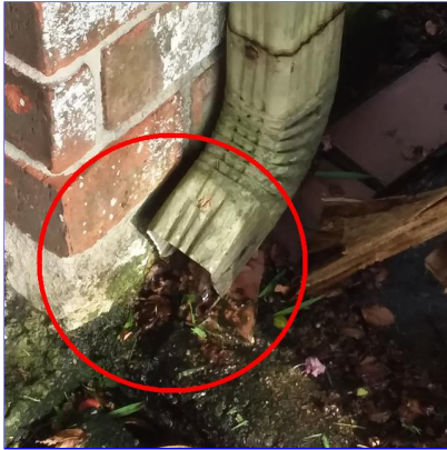
B. Item 4(Picture) Front of home
