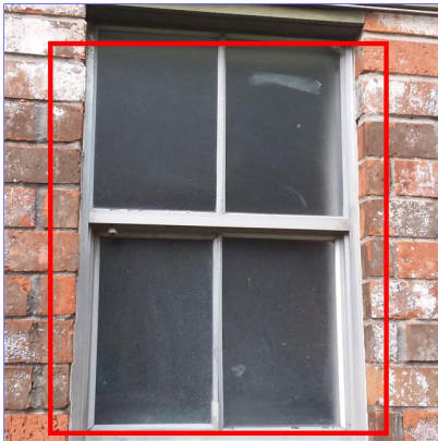
H. Item 7(Picture) Right side of home
