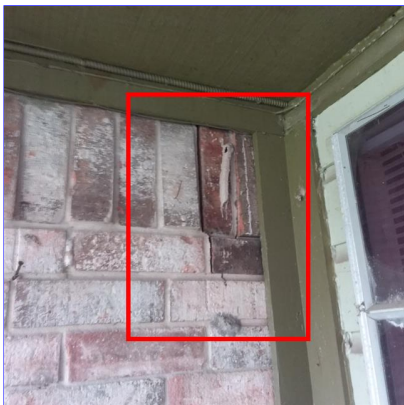
E. Item 43(Picture) Left rear of home
