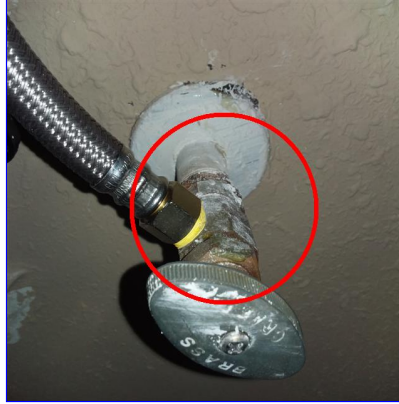
A. Item 4(Picture) Hall bath sink
