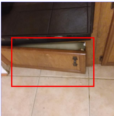
I. Item 3(Picture) Front of kitchen
