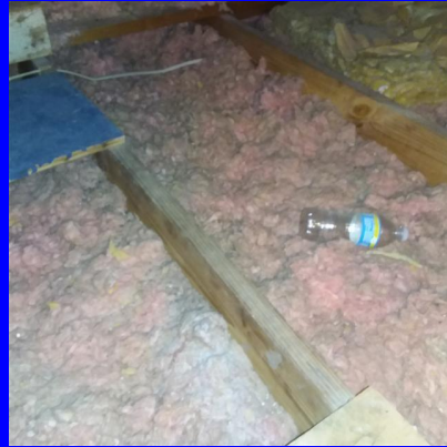
5 inches of blown insulation
