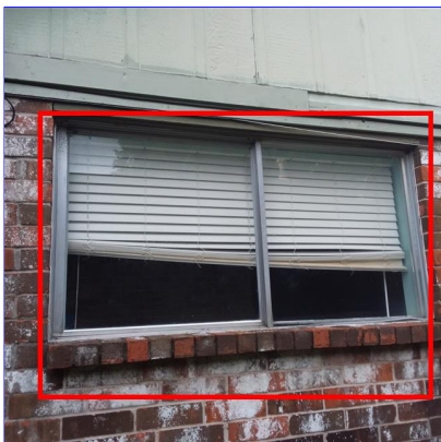
H. Item 10(Picture) Right side of home
