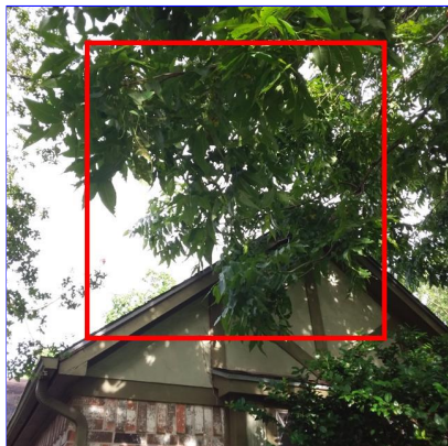
C. Item 1(Picture) Front of home
