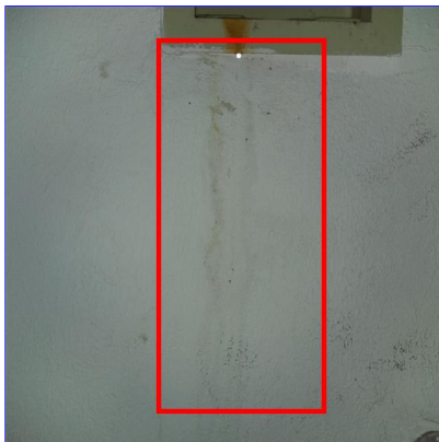
E. Item 30(Picture) Rear of washer/dryer room
