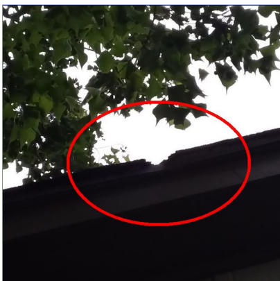
C. Item 7(Picture) Rear of home
