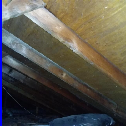
Roof structure stick built
