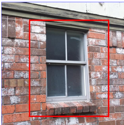
H. Item 11(Picture) Right side of home
