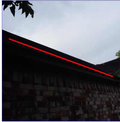
B. Item 3(Picture) Front right side of home
