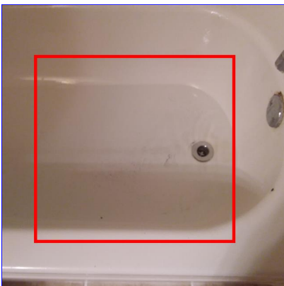
B. Item 2(Picture) Hall bath
