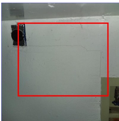
E. Item 20(Picture) Rear of washer/dryer room
