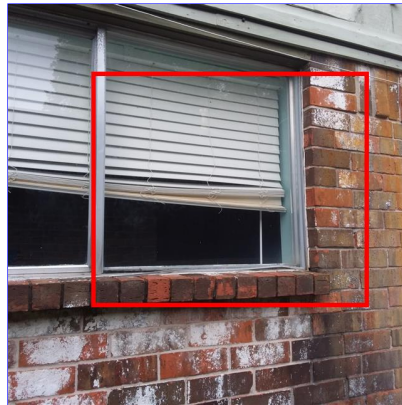
H. Item 8(Picture) Right side of home
