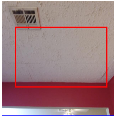
F. Item 10(Picture) Right side of sunroom
