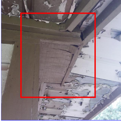
E. Item 5(Picture) Left rear of home
