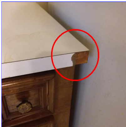
I. Item 7(Picture) Front of kitchen
