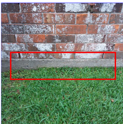
A. Item 2(Picture) Right side of home
