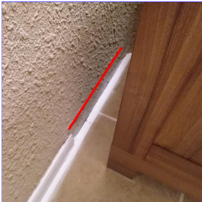
E. Item 34(Picture) Hall bath
