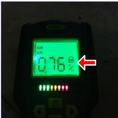
E. Item 29(Picture) Rear of washer/dryer room
