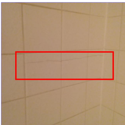
E. Item 35(Picture) Hall bath
