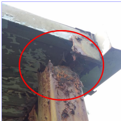
K. Item 4(Picture) Rear of home
