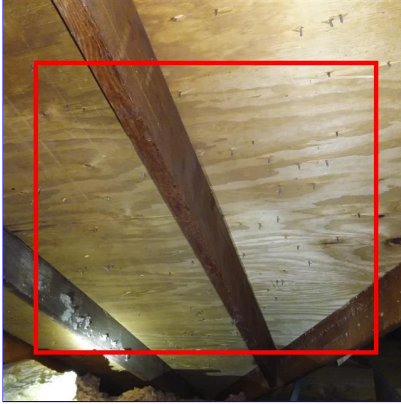
D. Item 3(Picture) Attic
