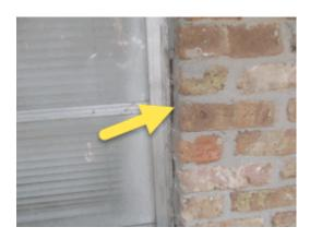
Stair step pattern of brick/mortar separation was found, a condition normally associated with foundation movement.
