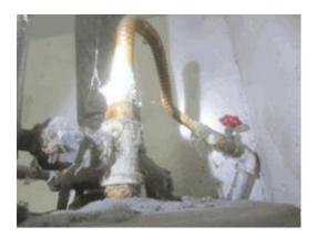
Flue vent pipe was found damaged/detached at the attic space (Hazardous condition).
