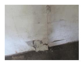
Interior wall cracks were observed at various locations. Also separation was observed where interior walls intersect. Settlement appears to be the cause.
