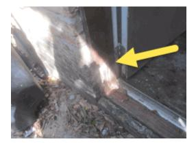
Separation was observed at the garage trim board & garage exterior door, a condition normally associated with foundation movement.
