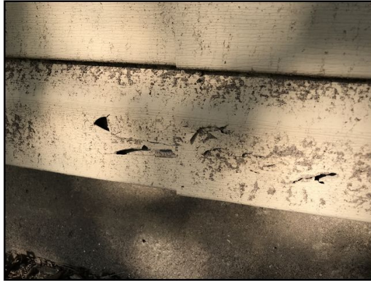
Potential rodent entry; south side of home at the soffit.
