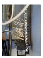
The grommet is missing around the metal knock-outs. Most of the supply wires are bundled where they go out of the main panel, this is common on most older homes but is not proper per current electrical standards.
