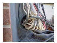
Also, there were breakers which appeared to serve a single conductor, indicating conductors may be connected to 240-volt circuits (red and black); trip ties are needed.
