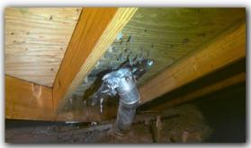
**NOTE:** I recommend the dryer exhaust be cleaned at a minimum of once per year to prevent clogs that could result in decreased efficiency, excessive appliance wear, and the possibility of a fire hazard. Functioning as designed at the time of the inspection.
