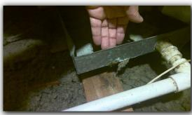
**REPAIR ITEM:** According to TREC standards A/C units should have a minimum of a 14 degree differential between supply. I recommend evaluation and repair by a licensed HVAC technician.
