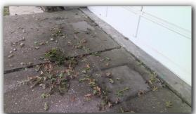
**REPAIR ITEM:** There were corner pops on the structure. Corner pops are not an uncommon occurrence on concrete slab foundations and typically have no bearing on the function of the foundation. I do recommend they be sealed with hydraulic cement to prevent the possibility of moisture and/or pest penetration.
