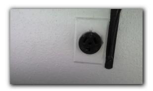
**REPAIR ITEM:** According to current standards all bathroom sinks must have a GFCI protected outlet within 3' of a sink. The left side sink in the primary bathroom did not meet this standard.
