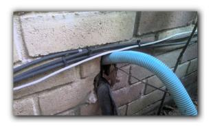
**REPAIR ITEM:** The suction line insulation on the exterior compressor unit needed to be repaired or replaced.
