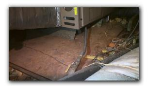
**SAFETY CONCERN:** A flexible gas line was penetrating through the appliance wall.
