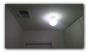
**REPAIR ITEM:** The mechanical exhaust fans were venting into the attic. They should vent to the exterior of the building envelope.
