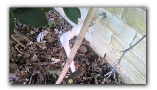
**REPAIR ITEM:** An anti-siphon device was missing on hose bibs.
