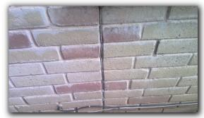
**REPAIR ITEM:** There were cracks in the brick and/or mortar. This may have been the result of a foundation or structural issue. I recommend sealing the cracks to prevent possible water and/or pest intrusion that could eventually damage the components behind the brick.
