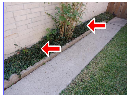
Right side of foundation
