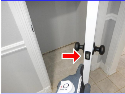
Closet door locking assembly
