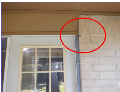
Rear brick wall
