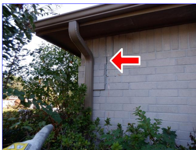
Front brick wall
