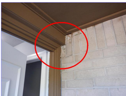
Entrance brick wall
