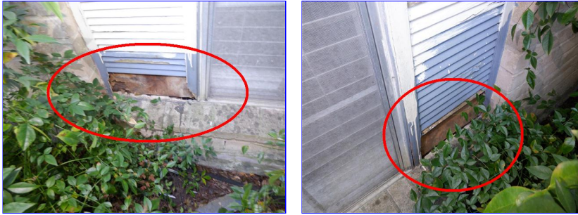
Front window walls
