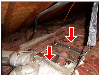
Attic insulation depleted
