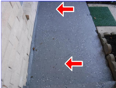
Front entrance foundation
