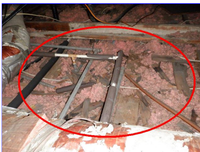
Attic insulation depleted
