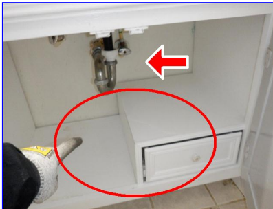
Master bathroom sink base
