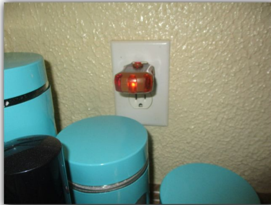
OUTLET REAR WALL OF KITCHEN COUNTERTOP IS REVERSE POLARIZED
