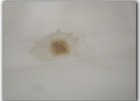
SURFACE MASTER TUB HAS BEEN PATCHED
