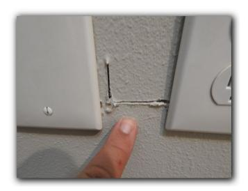
CALKING/GROUT AND SOME PAINT DEFICIENCIES IN THE BATHROOMS, DOOR FRAME/BASE BOARDS TRIM, AND THE CLOSET HANGER RODS NEED PAINTING
