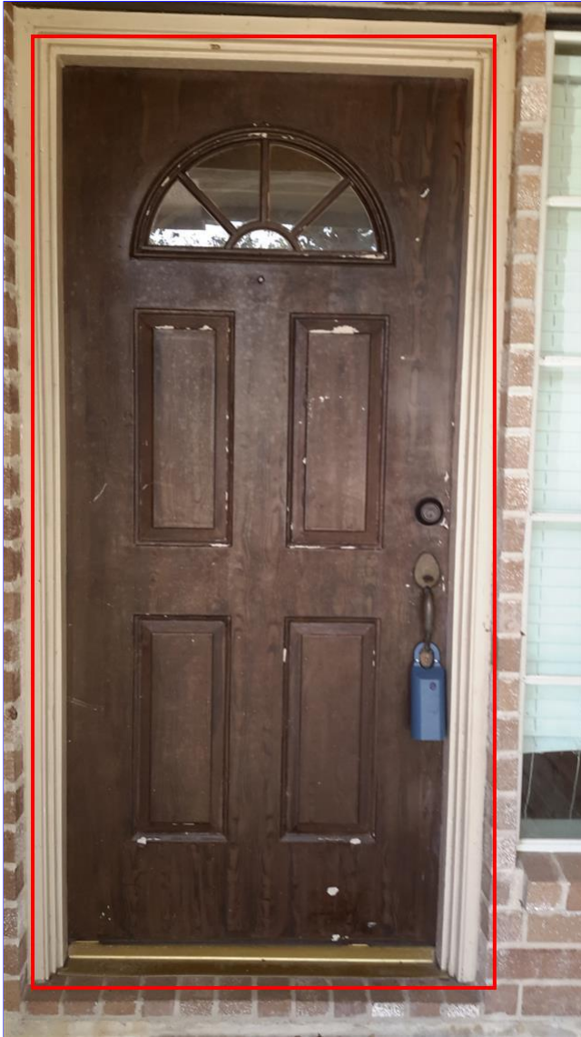
G. Item 1(Picture) front door
