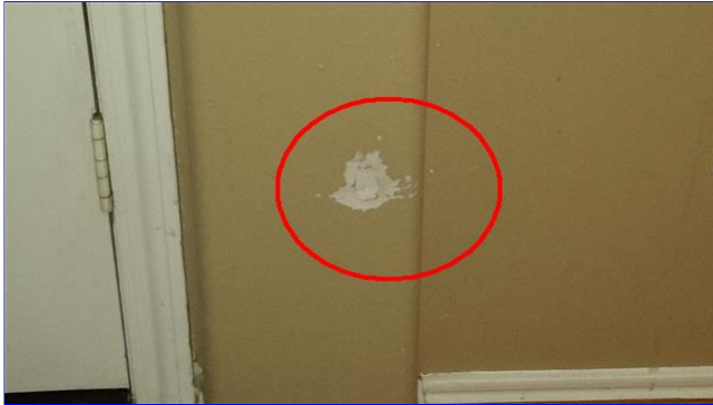
E. Item 19(Picture) entry hallway
