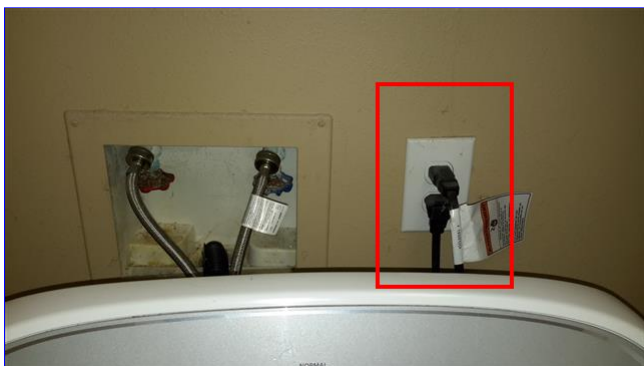
B. Item 1(Picture) laundry room
