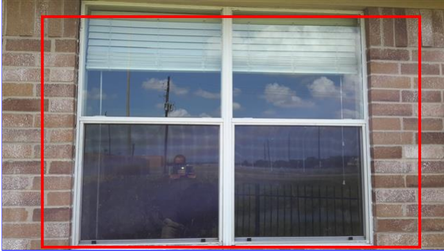
H. Item 3(Picture) right side of home
