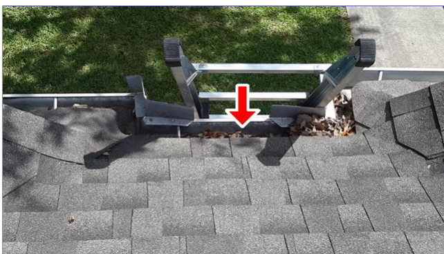
B. Item 3(Picture) front of home
