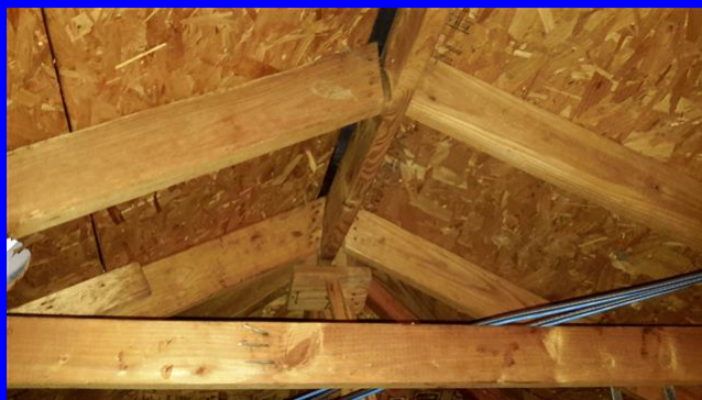
stick built no radiant barrier
