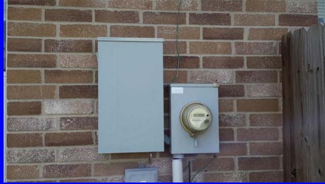
Meter box and breaker box right side of home
