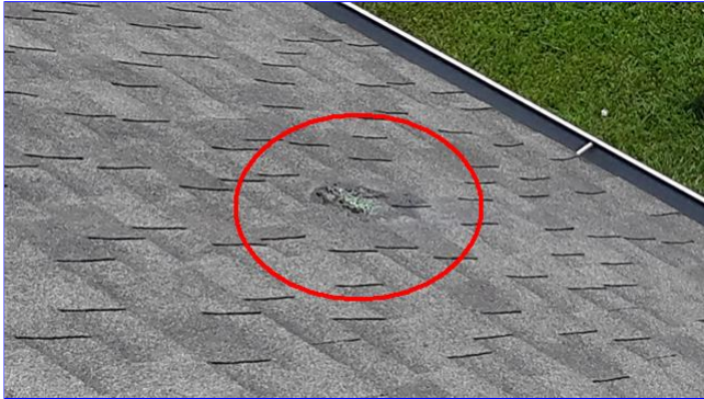
C. Item 8(Picture) left side of home
