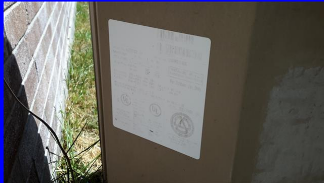
data plate faded MFD not listed
