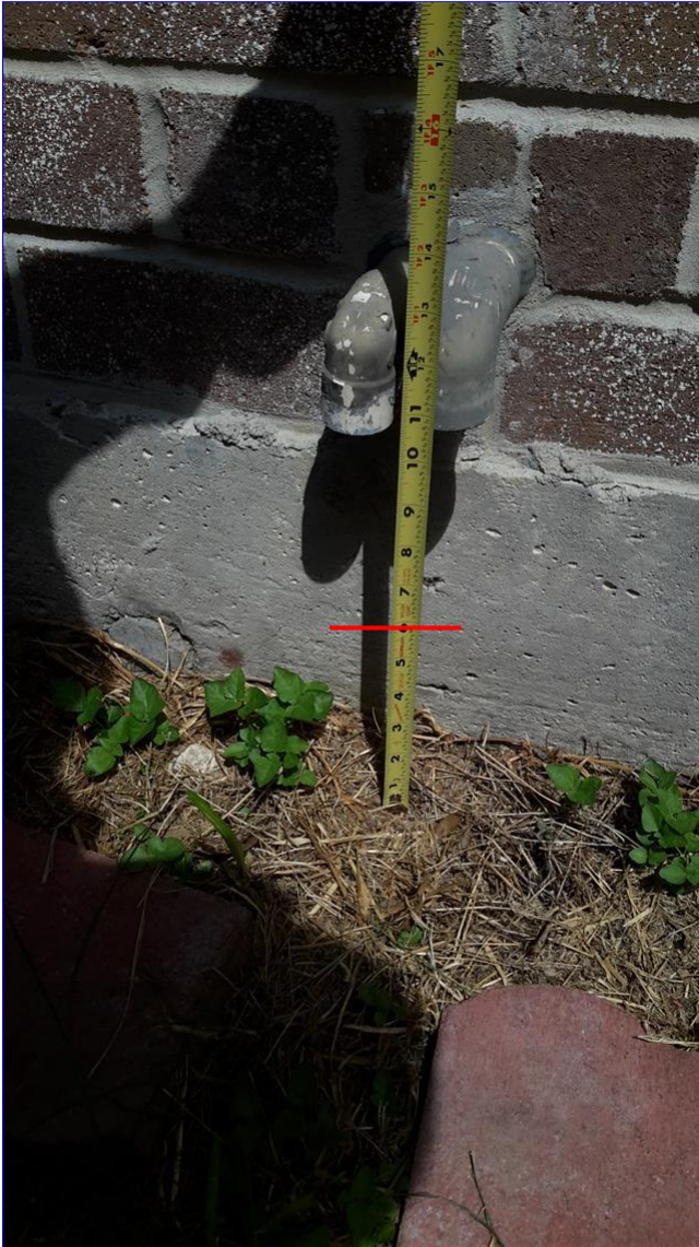
C. Item 2(Picture) left side of home
