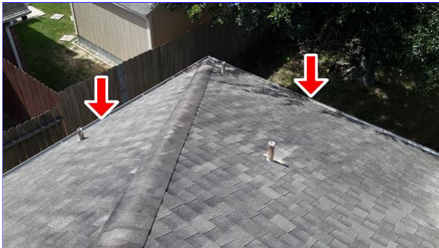
B. Item 1(Picture) left side and rear of home.
