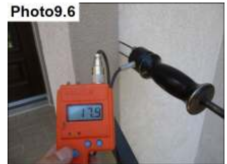
Moisture Probe/ Right Side Of Column Below Balcony
