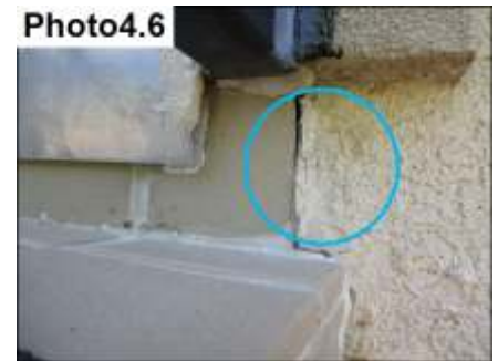
Balcony Flashing Sealants/ Seal
