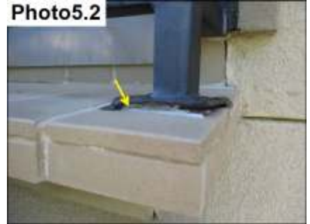
Penetration Sealants/ Seal
