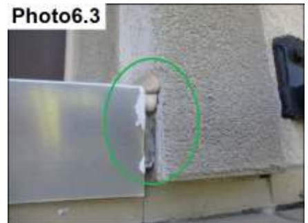
Door Trim/Threshold Sealants/ Seal
