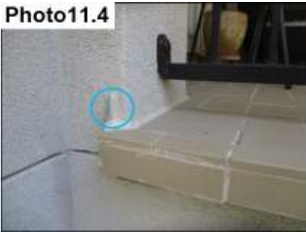
Balcony Flashing Sealants/ Seal
