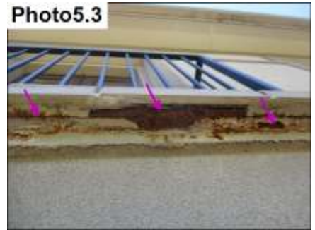
Penetration Sealants/ Seal
