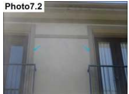
Photo7.2 Different Color Sealants/ Touch Up
