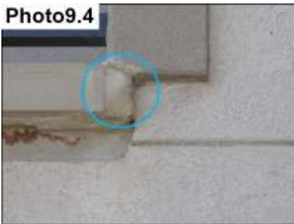
Balcony Flashing Sealants/ Seal
