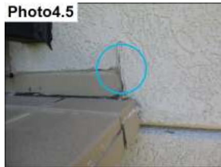
Balcony Flashing Sealants/ Seal
