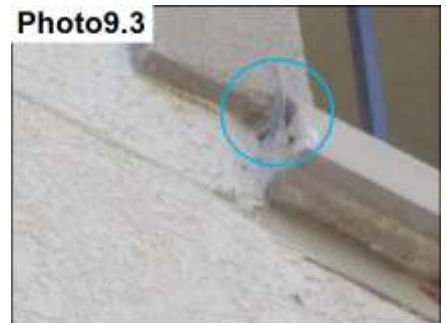
Balcony Flashing Sealants/ Seal
