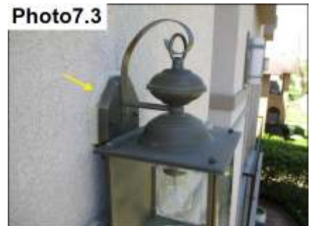
Photo7.3 Penetration Sealants/ Maintain
