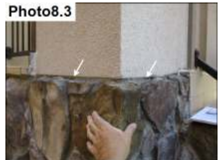
Stone/Stucco Termination Sealants/ Seal
