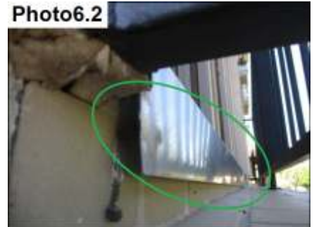
Door Trim/Threshold Sealants/ Seal
