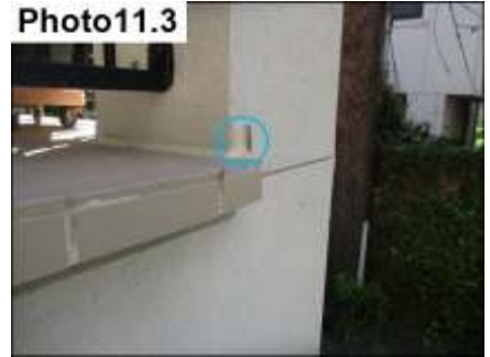
Balcony Flashing Sealants/ Seal
