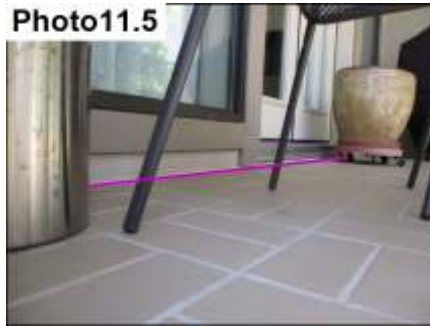
Balcony/Stucco Termination Properly Sealed/ Positive Detail
