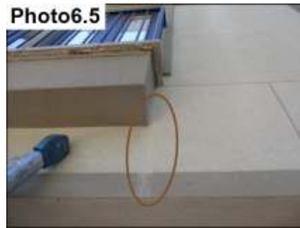
Efflorescence Noted
