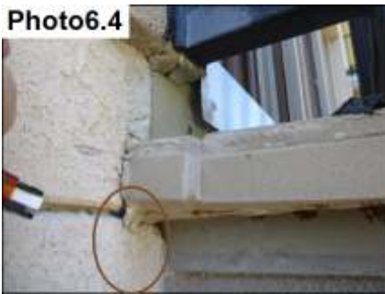
Efflorescence Noted
