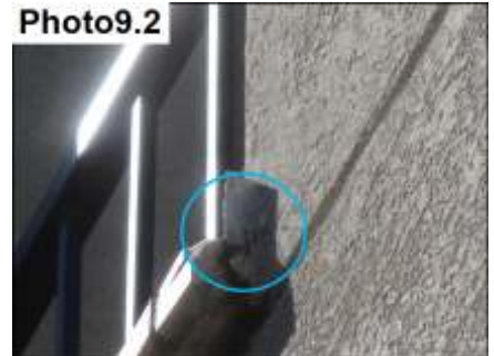
Balcony Flashing Sealants/ Seal
