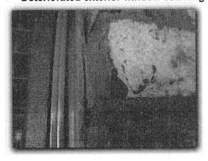
Missing/broken (or not properly sized) 4 window screens, sticky window operations, damaged springs in window tracks noted in the house.
