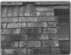
The right side of the brick veneer wall was discolored (rusty color), cause by A/C condensate drips from roof eave.
