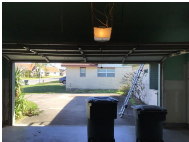
General Photos of Dryer Exhaust Systems:
