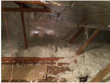
Approximate Average Depth of Insulation: 12 Inches
