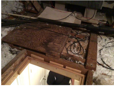
Approximate Average Depth of Insulation: 12 Inches
