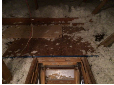
Approximate Average Depth of Insulation: 12 Inches
