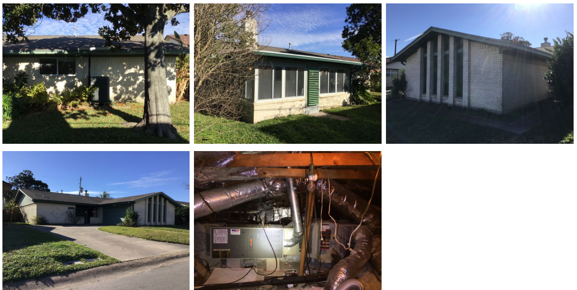
General Photos of Roof Covering:
