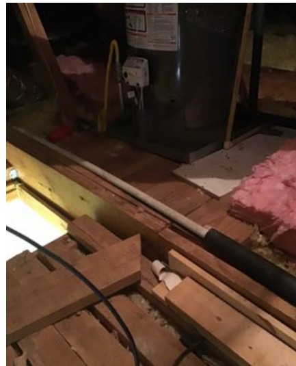
Condensation line is not fully wrapped with insulation
