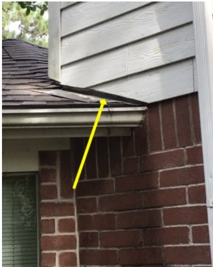
Kick out flashing is missing. This would prevent water shedding from the roof onto the brick veneer
