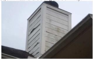
The sealant at most penetrations of the house is deteriorated or gaps in material. All penetrations and openings around the exterior should be properly sealed with caulk, screen mesh, expanding foam or mortar as needed to keep out moisture and unwanted pests (Do not seal up weep holes where the brick meets the slab).
