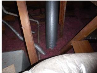
There is evidence of rodents in the attic by trampled, uneven insulation and of rodent droppings. Recommend quarterly pest control and eradication by a licensed professional.
