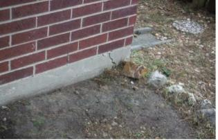
The foundation cable ends are exposed which over time can rust and weaken the strength of the cables possibly causing foundation problems/repairs in the future if the current condition is not repaired. Remove the rust from the cable and cover with rust inhibitor primer and seal with a high strength non-shrink grout.
