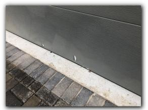
All exterior wall penetrations (electrical panels, electrical disconnects, light fixtures, etc.) and openings (expansion joints, windows, door thresholds, etc.) should be sealed with an approved material to prevent water penetrations into the wall cavities. Properly sealed exterior veneers help provide a barrier against the weather, insects, and enable environmental control of the interior spaces.
