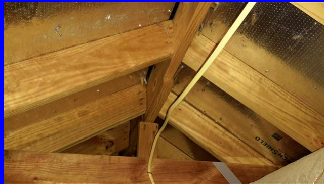
Roof structure from the attic
