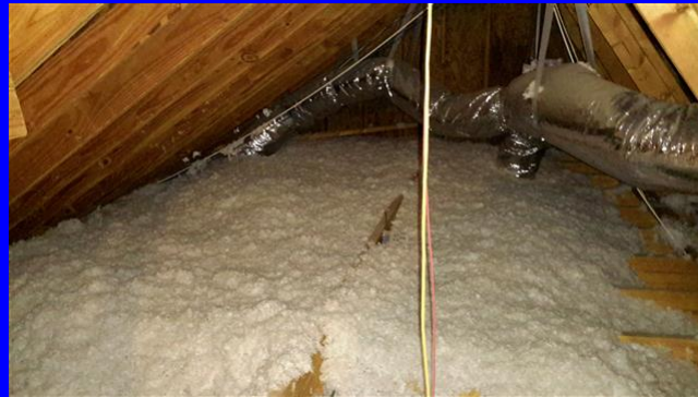
approximately 12 inches of insulation in the attic
