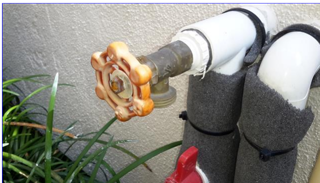
A. Item 2(Picture) at main water entrance
