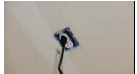
Missing outlet/switch cover plates in the garage/shop should be replaced.
