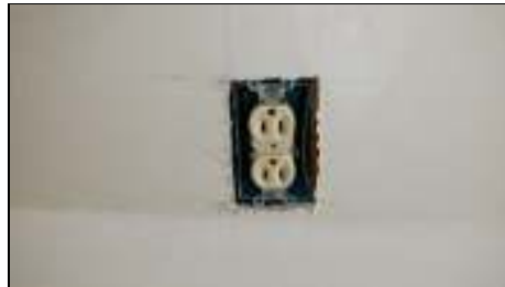
Missing outlet/switch cover plates in the garage/shop should be replaced.
