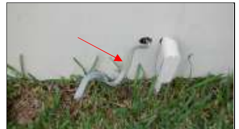
Abandoned wiring at the rear of the garage should be appropriately terminated.
