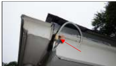
Abandoned wiring at the rear of the garage should be appropriately terminated.
