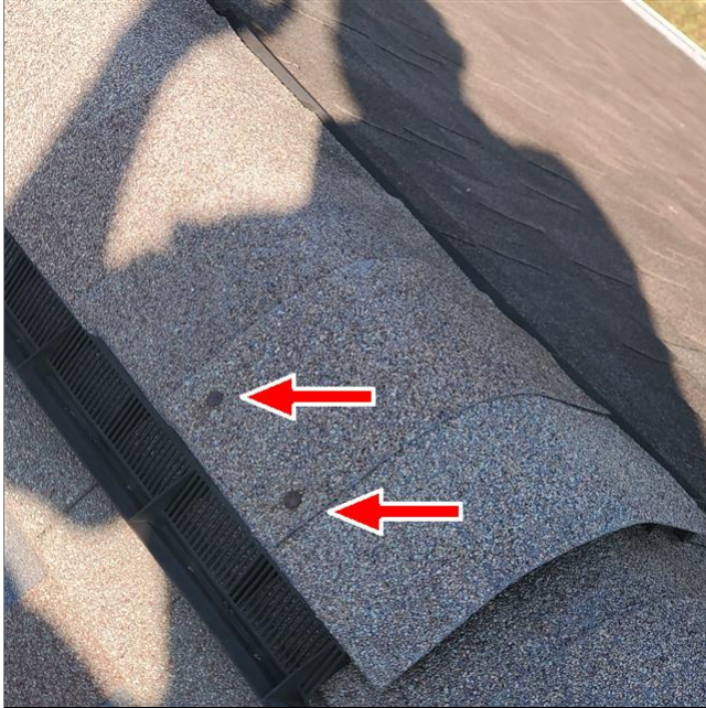
C. Item 7(Picture) Photo of two of the unsealed nails.
