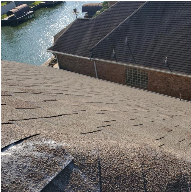
C. Item 3(Picture) Roof overview.
