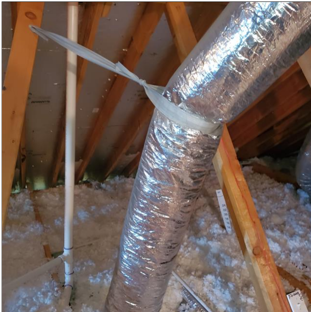
F. Item 3(Picture) There was no visibly damaged insulation.
