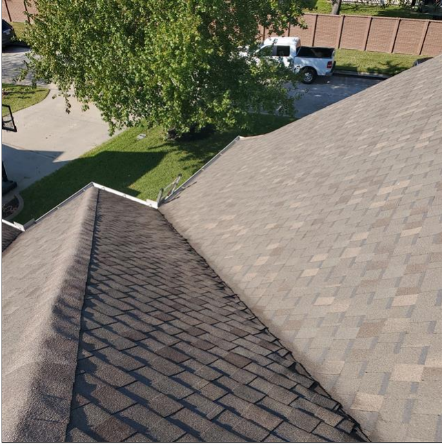
C. Item 1(Picture) Roof overview.
