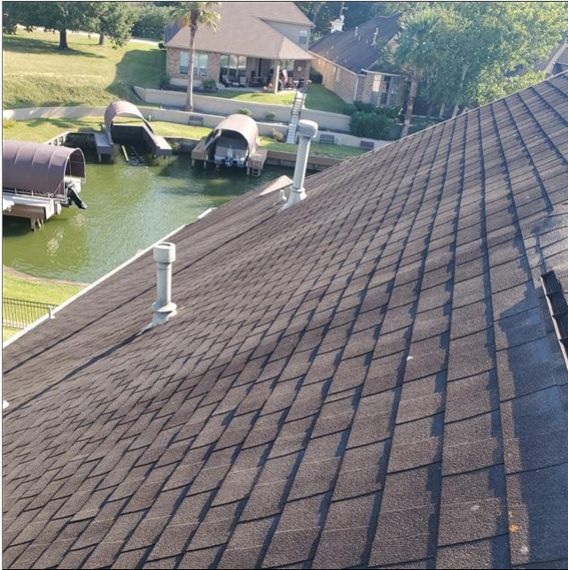
C. Item 2(Picture) Roof overview.
