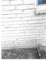
The left photo above is the crack in the front bedroom slab. The center photo show the continuation of the crack toward the hall. The right photo is the exterior wall on the back side of the house that had a hairline crack in the brick veneer only. It was noted that there were no cracks in the bedroom slab in the bedroom on the other side of this exterior wall.
