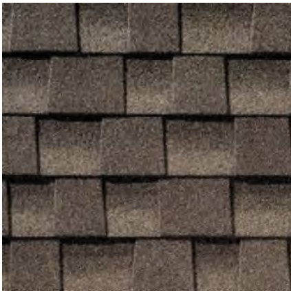
Roof. Weathered Wood Per Community Guidelines
