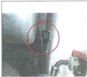
Ungrounded outlet and not on GFCI on kitchen counter downstairs
