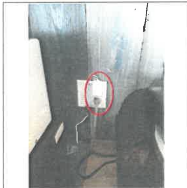
Ungrounded outlet and not on GFCI on kitchen counter downstairs
