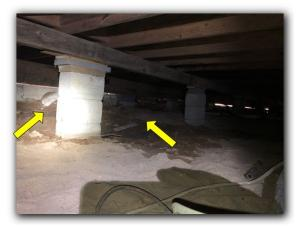
There was no apparent evidence, in my opinion, that would indicate the presence of major foundation deformities, excessive settlement distress conditions, or significant deficiencies in the foundation. Interior and exterior stress indicators showed little effects of adverse performance. The foundation appeared to be performing at the time of the inspection without the obvious need of immediate remedial leveling and was providing adequate support for the structure.
