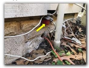
• There was no electrical receptacle installed on the exterior wall of the front entry area. As per IRC 3901.7, there is to be an accessible electrical receptacle at the front and rear of the dwelling.
