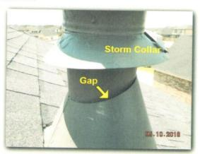
X: Daylight around the water heater exhaust flue was noted from inside the attic. This gap might allow water penetration and should be sealed above the roof.
