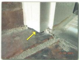
X: The garage vehicle door casings are angle cut to allow painting in order to prevent material breakdown. The angle cuts were not fully painted.
