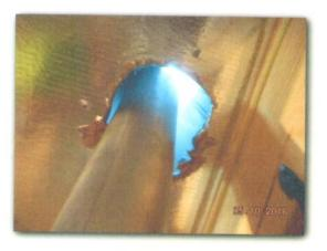
X: The water heater flue vent is not properly secured in the attic space. It should be secured to the adjacent wood rafters with a metal strap, to prevent any contact with combustible materials (wood roof sheathing), which may start a fire. This is a safety hazard.
