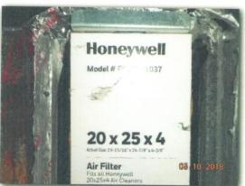
X: Dirty media filter was noted in line with the air handler in the attic. It should be changed regularly for an efficient operation of the cooling/heating equipment. Dirty media filters can cause dirty coils at the evaporator which can have a negative effect on the performance of the A/C system.
