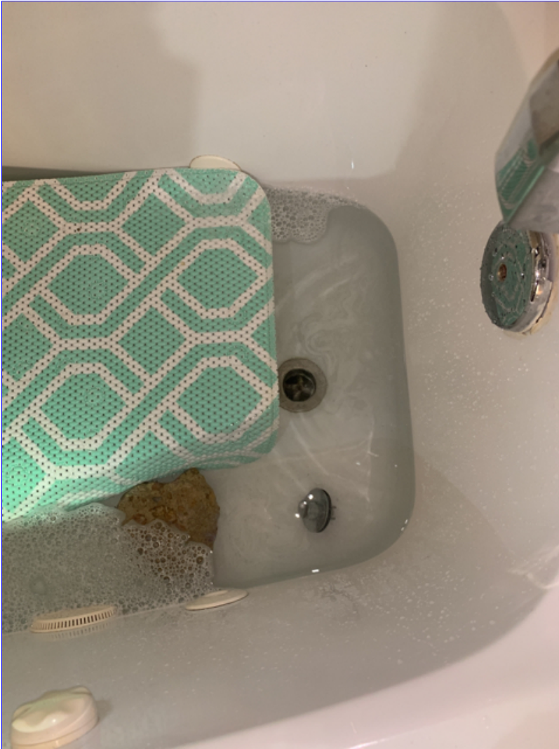
B. Photo 1(Picture) The whirlpool bath is very slow to drain.
