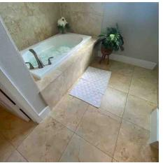
• The spa tub would not shut off with the switch. I had to trip the GFCI for the tub to stop the motor. Recommend repair by qualified plumbing contractor.
