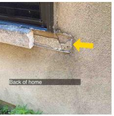
• The exterior walls of this house appear to be standard wood frame construction. The visible exterior is stucco and composite concrete veneer that has been installed over the wood framing. The interior walls are covered with drywall.
