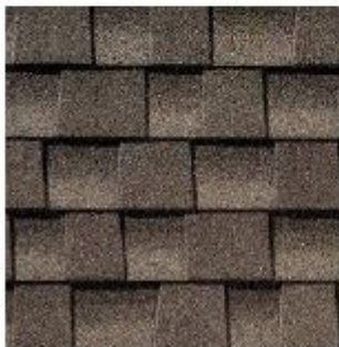
Roof. Weathered Wood Per Community Guidelines
