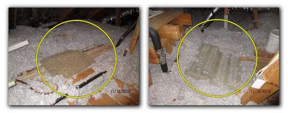
• Some of the soffit baffles in the attic area are loose and not properly secured. "Baffles" should be installed along these areas to hold back insulation and allow for free movement of air within the roof space. It is recommended that these conditions be further investigated and improved where necessary.
