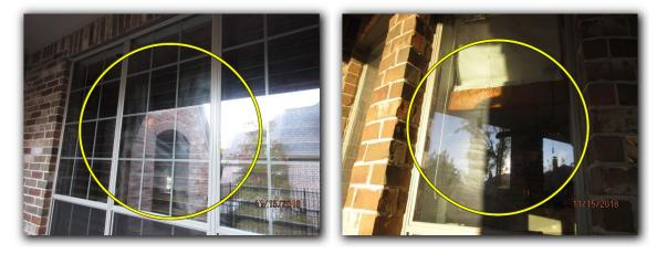
• The frame guide balances are loose/damaged and not properly secured along some of the windows (Breakfast Room). It is recommended that the guide balances at all windows be checked by a qualified company to ensure that they are installed properly and allowing for normal operation.
