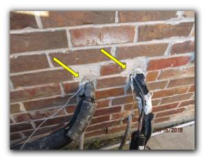
• Damaged/missing insulation was noted along the refrigerant lines at the A/C condenser unit located outside.
