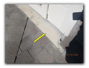
• Some of the flashing is loose and not properly secured to the roofing material. These conditions should be repaired to reduce the risk of water penetration and promote proper water drainage from the roof covering material.
