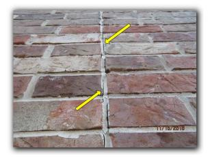
• The caulking was noted missing or not installed along some of the vertical siding junctions. These areas should be properly sealed to reduce the risk of moisture penetration.
