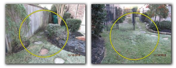
• The soil level at the foundation is too high (Various Locations). Under current building standards/practices the exposed height of the exterior perimeter beam of the foundation should be maintained a minimum of 4 inches above the soil level for concrete or masonry type siding, and a minimum of 6 inches above the soil level for wood type siding.
