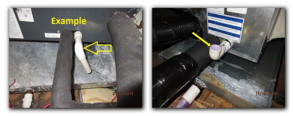
• Some of the insulation joints along the A/C refrigerant lines in the attic area are not sealed properly. Condensation forms on the exposed copper refrigerant lines when the A/C system is operating. All of the insulation joints along the refrigerant line should be properly sealed to reduce the risk of water damage to the structure.
