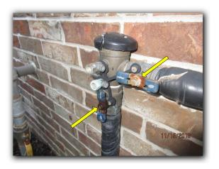
• The bell cap to the vacuum breaker appeared to be damaged at the time of inspection. It is recommended that this condition be further investigated and repairs undertaken as necessary.
