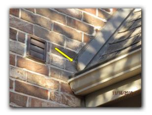
• All exposed nail heads along the roof flashing and roof jack flanges should be properly sealed to reduce the risk of water penetration.
