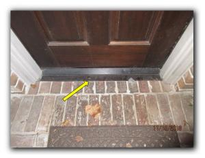
• As preventative measures, the frame and threshold junctions along all exterior entry doors should be properly sealed to reduce the risk of water penetration and insect activity (Various Exterior Doors). (See Exhibit Below)
