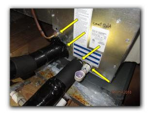
• The drain line to the over-flow opening along the evaporator cabinet does not terminate properly into the safety pan. This condition requires further investigation and repairs undertaken as necessary to reduce the risk of water damage to the structure.
