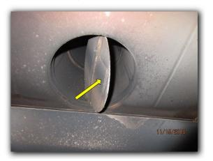
• Missing paint was noted to the metal chimney cap. As preventative measures, it is recommended the metal chimney cap be painted to reduce the risk of corrosion/degradation from weather conditions.
