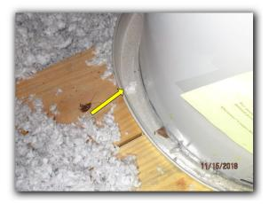
• The auxiliary (safety) drain pan installed below the water heater unit appears to be off-center of the unit and not properly installed below the tank drain valve. This condition requires further investigation and repairs undertaken as/if needed to reduce the risk of water damage in the event of a leak.
