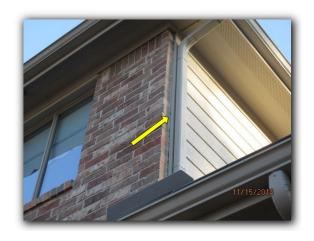
• The following components/items mounted, entering or terminating along the exterior walls should be properly sealed at the wall junctions to reduce the risk of air leakage, water penetration and insect activity (Pool Equipment Panel Boxes).
