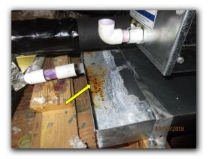
• The openings in the evaporator coil cabinet where the refrigerant lines enter should be sealed properly to reduce the risk of air leaks.
