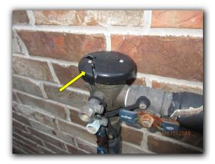
• The sprinkler system was found to be inoperative at the time of inspection. The system did not respond when the controller was actuated. The system appears to be winterized (water supply turned off). This condition should be further investigated and repairs undertaken as necessary to ensure that the system works properly.
