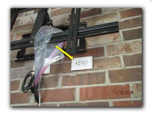
Some of the outlets are not functioning at the time of inspection (Left Side of House). These outlets and their circuits require further investigation and repairs undertaken as necessary.
