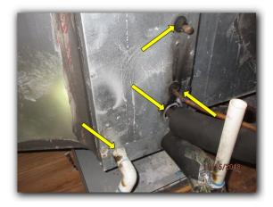
• Some of the insulation joints along the A/C refrigerant lines in the attic area are not sealed properly. Condensation forms on the exposed copper refrigerant lines when the A/C system is operating. All of the insulation joints along the refrigerant line should be properly sealed to reduce the risk of water damage to the structure.
