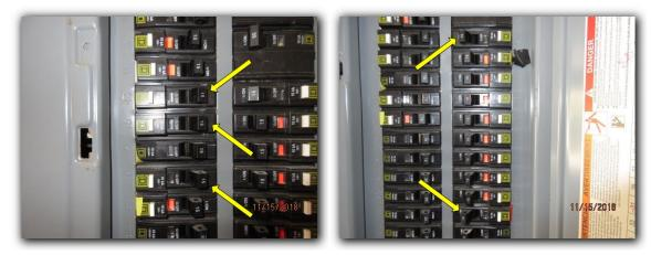
• The white wire to the 220/240 volt circuit is not marked as a hot wire. Under current building standards/practices, the white wire should be marked with black or red to indicate that it is a hot and not a neutral.
