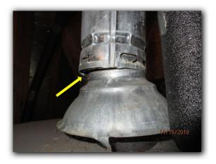
• The vent pipe serving the water heater does not have safe clearance from combustible materials. This condition should be improved for safety reasons. Exhaust flues require a minimum 1" clearance from combustibles.
