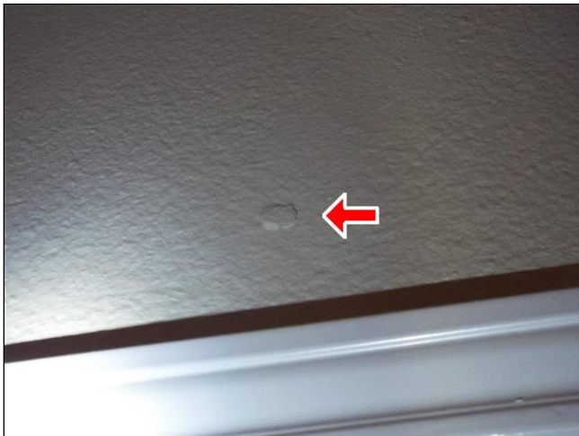
F. Item 26(Picture) Nail popping appears over front door trim frame.
