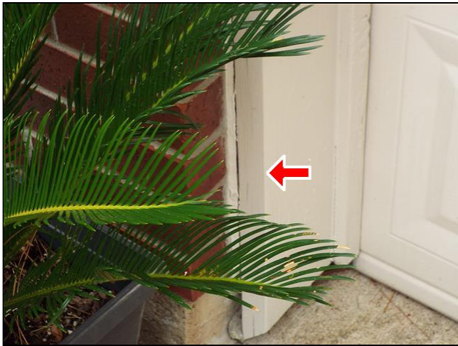
F. Item 1(Picture) Sealing is needed around the perimeter of garage door trim board.
