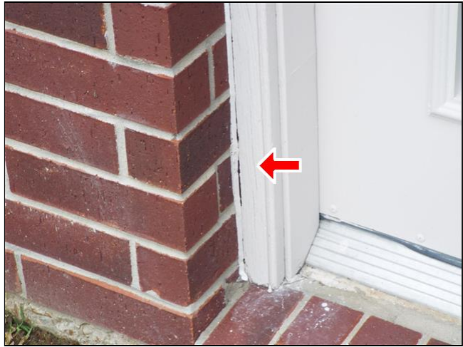
F. Item 14(Picture) Caulking and painting is needed around the wood frame at rear entrance. Damaged wood near threshold plate is in need of repair.
