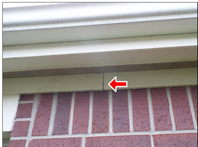
F. Item 12(Picture) Seams along fascia board and brick fascia boards are in need of sealing and painting.
