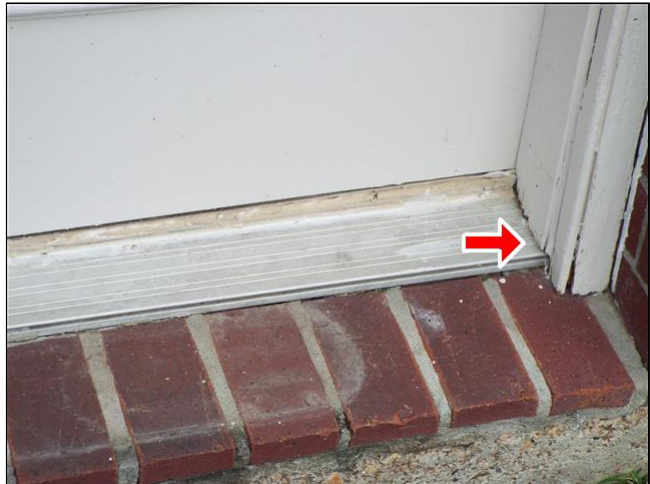
F. Item 16(Picture) Caulking and painting is needed around the wood frame at rear entrance. Damaged wood near threshold plate is in need of repair.
