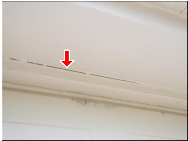
F. Item 2(Picture) Sealing is needed around the perimeter of garage door trim board.
