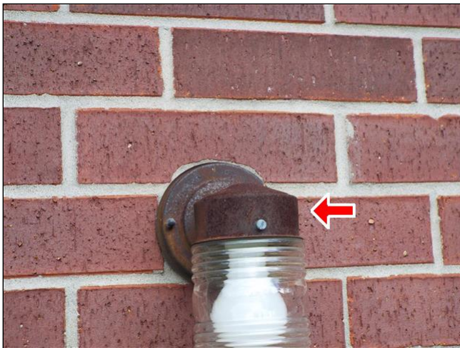
B. Item 1(Picture) Rear light fixture is rusted and is in need of repair or replacing.
