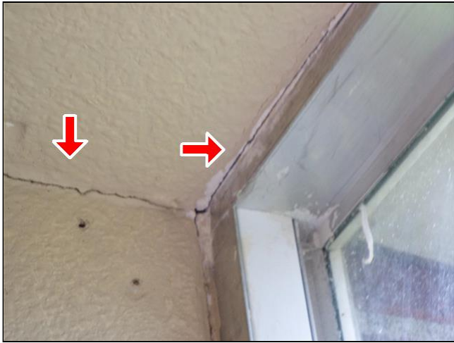
H. Item 5(Picture) Caulking is needed in the corner of window interior.
