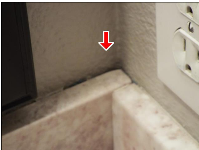
F. Item 30(Picture) Sealing is needed in corners and seams in bathroom.
