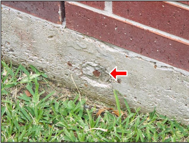
A. Item 5(Picture) Post tension holes along the foundation perimeter needs filling.
