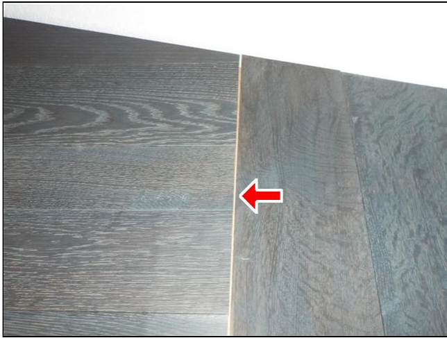
F. Item 34(Picture) Wood over fire place is in need of securing.
