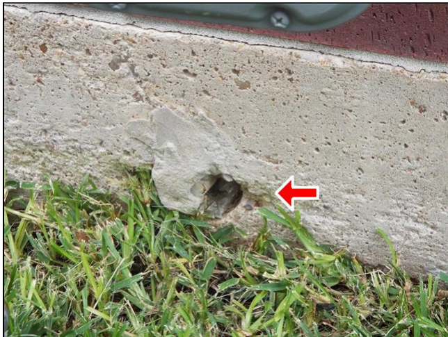
A. Item 1(Picture) Post tension holes along the foundation perimeter needs filling.
