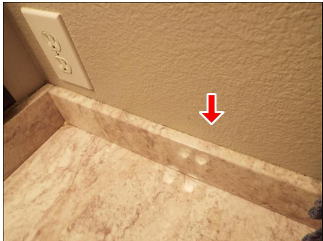
F. Item 27(Picture) Sealing is needed in corners and seams in bathroom.
