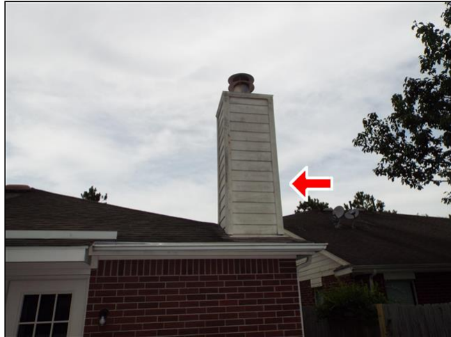
J. Item 2(Picture) Chimney is in need of repair and painting.
