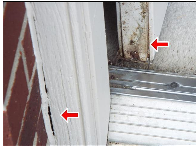
G. Item 4(Picture) Rear door has soft wood at the bottom,
