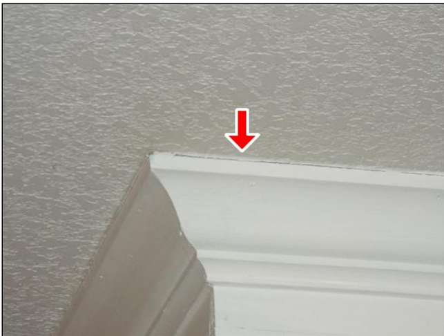
E. Item 3(Picture) Repair is needed around molding inside at ceiling between living room and kitchen.
