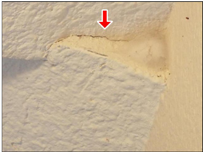
F. Item 41(Picture) Crack in ceiling corner near master bedroom entry is in need of repair.
