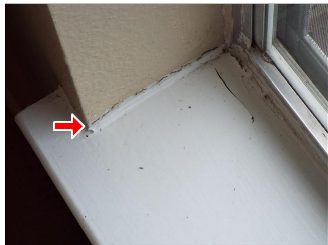
H. Item 4(Picture) Caulking is needed in corners of window sills.
