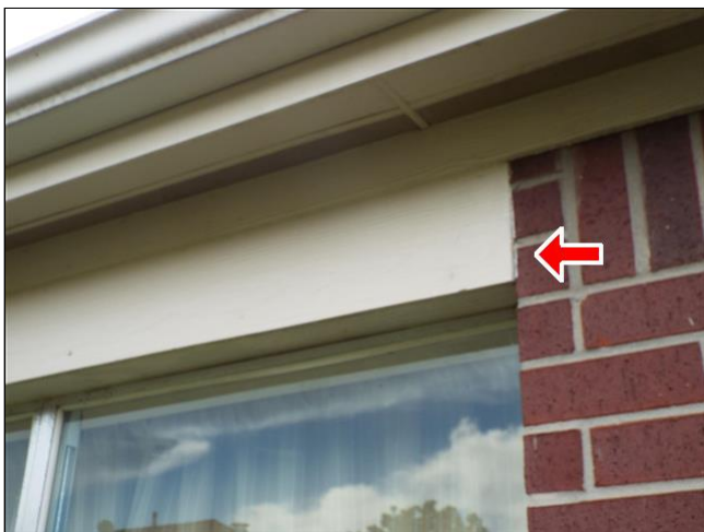
F. Item 11(Picture) The corner of siding over windows are in need of repair.
