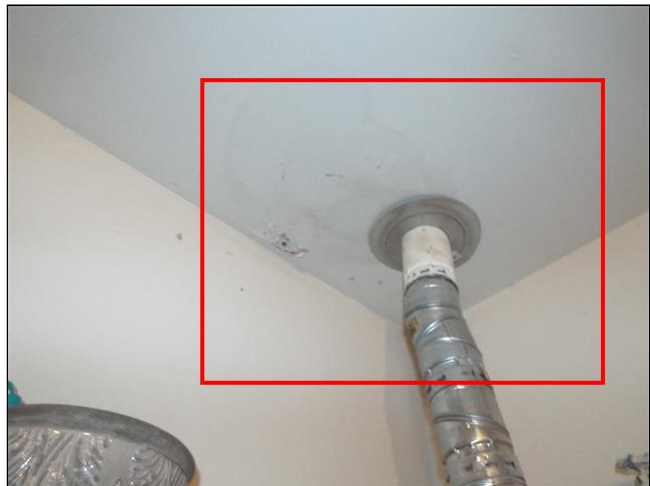
E. Item 4(Picture) Ceiling is in need of repair near water heater flue pipe. client would like to know have any repairs been made in area.
