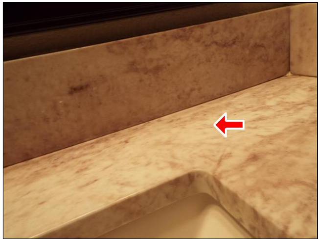
F. Item 29(Picture) Sealing is needed in corners and seams in bathroom.
