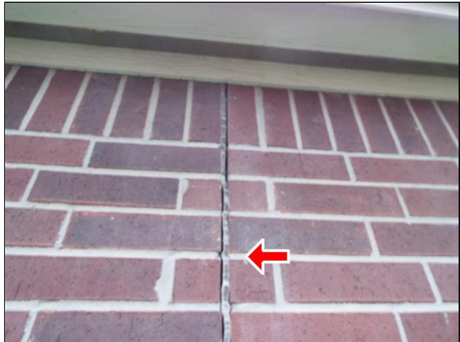
F. Item 20(Picture) Expansion joint is in need of caulking.
