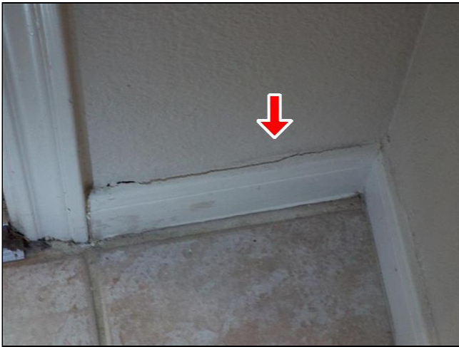
E. Item 1(Picture) Base board around front door is in need of repair.
