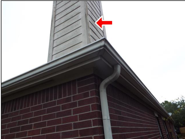
J. Item 1(Picture) Chimney is in need of repair and painting.
