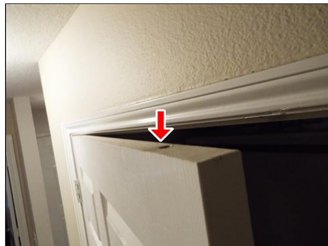
G. Item 2(Picture) Latching component is missing from utility closet door.
