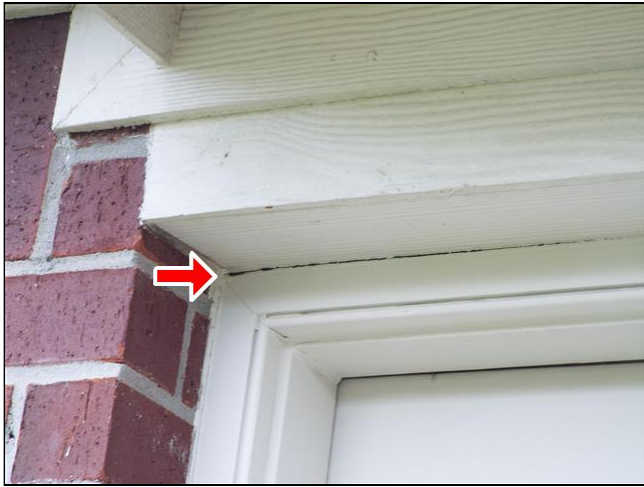
F. Item 13(Picture) Siding corners and seams are in need of sealing.
