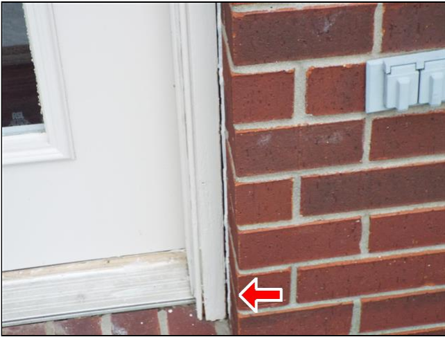
F. Item 17(Picture) Caulking and painting is needed around the wood frame at rear entrance. Damaged wood near threshold plate is in need of repair.
