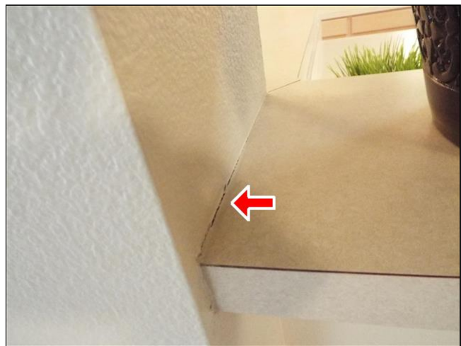
F. Item 37(Picture) The bar counter corner is in need of sealing.
