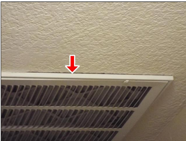
C. Item 1(Picture) Sealing is needed around return vent.
