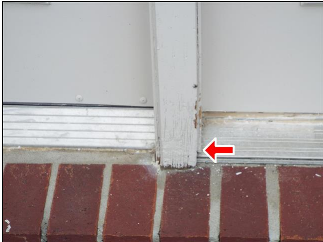
F. Item 15(Picture) Caulking and painting is needed around the wood frame at rear entrance. Damaged wood near threshold plate is in need of repair.
