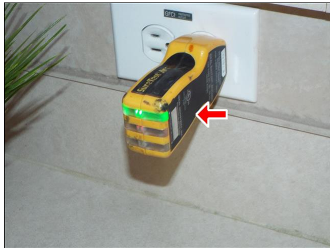
B. Item 2(Picture) Outlet along back splash should be checked for loose open ground.
