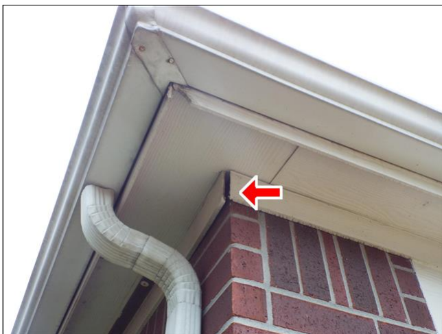
F. Item 5(Picture) Corners of brick fascia boards shows separation and seams are in need of sealing and painting. Repair is needed.
