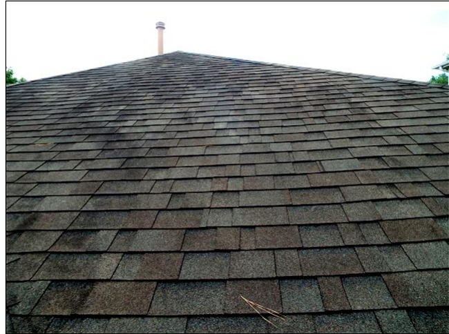
C. Item 2(Picture) Shingle edges appears to expose fibers.
