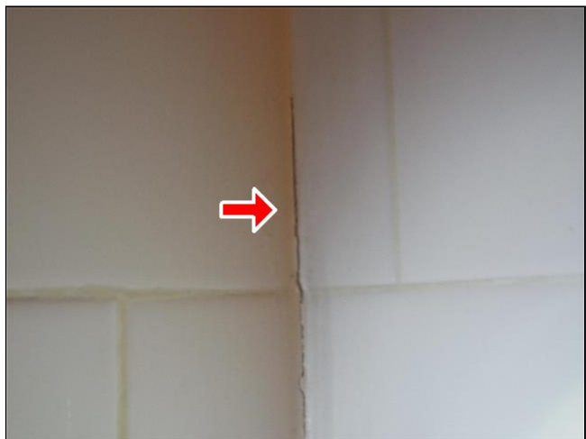
F. Item 31(Picture) Bath tub tile corner is in need of sealing.
