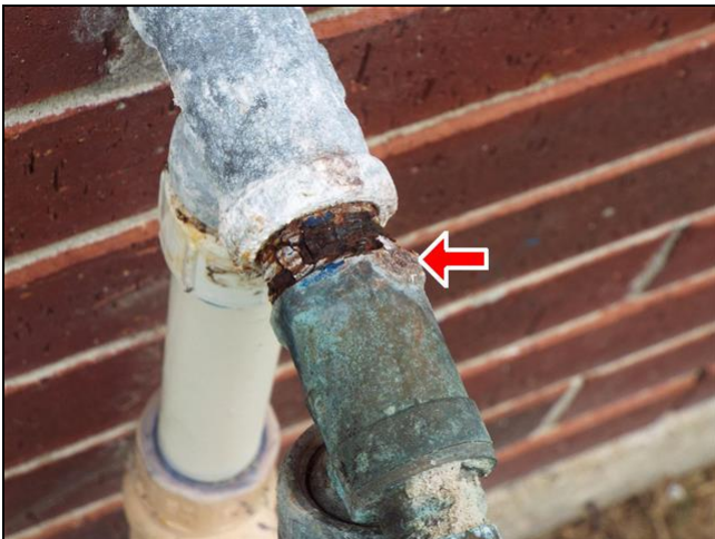
A. Item 1(Picture) plumbing nipple is rusted and needs to be repaired.
