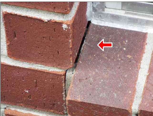
F. Item 21(Picture) The corner of brick under window area is in need of grout or some form of sealing.
