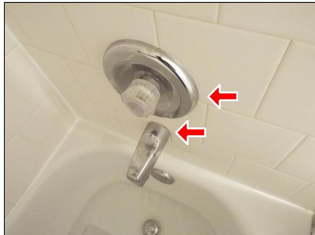
A. Item 2(Picture) Sealing is needed around fixtures.
