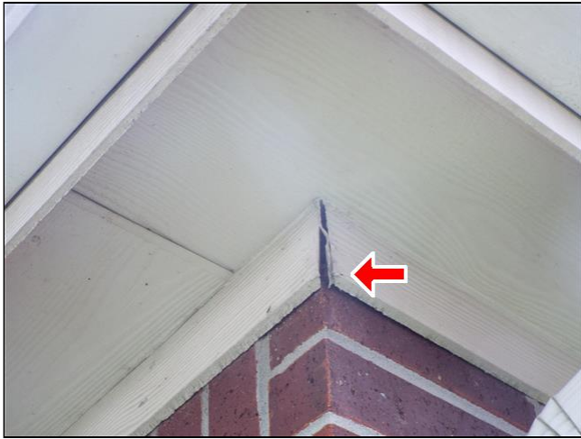
F. Item 23(Picture) Corners of brick fascia boards shows separation and seams are in need of sealing and painting. Repair is needed.
