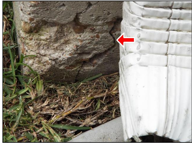
A. Item 6(Picture) Crack should be filled to prevent pest from entering structure.
