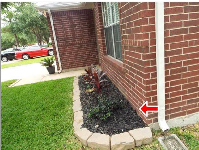
B. Item 3(Picture) Bedding appears to be covering foundation wall.
