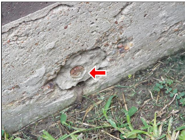
A. Item 3(Picture) Post tension holes along the foundation perimeter needs filling.
