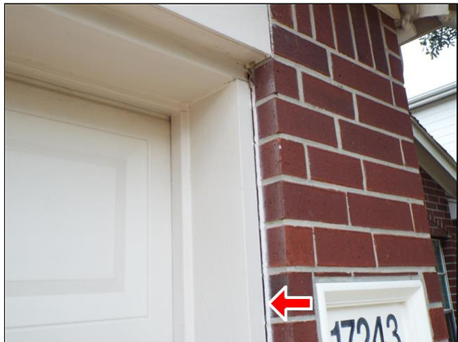
F. Item 4(Picture) Sealing is needed around the perimeter of garage door trim board.
