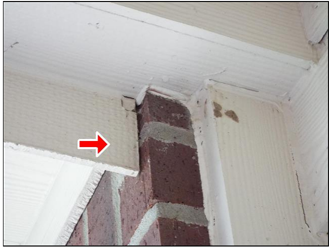
F. Item 24(Picture) Siding corners and seams are in need of sealing.
