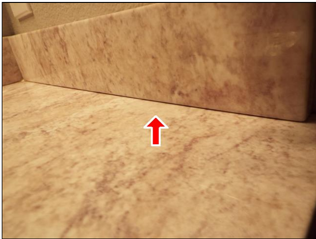
F. Item 28(Picture) Sealing is needed in corners and seams in bathroom.
