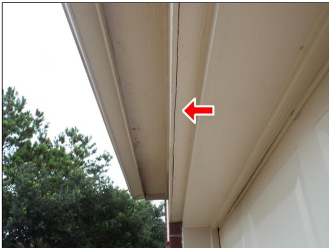
F. Item 3(Picture) Siding corners and seams are in need of sealing.
