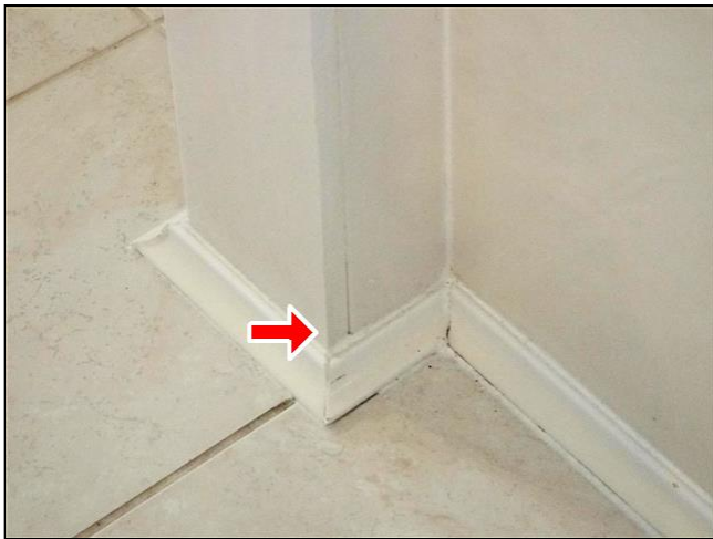
F. Item 40(Picture) Sealing is needed around base board.
