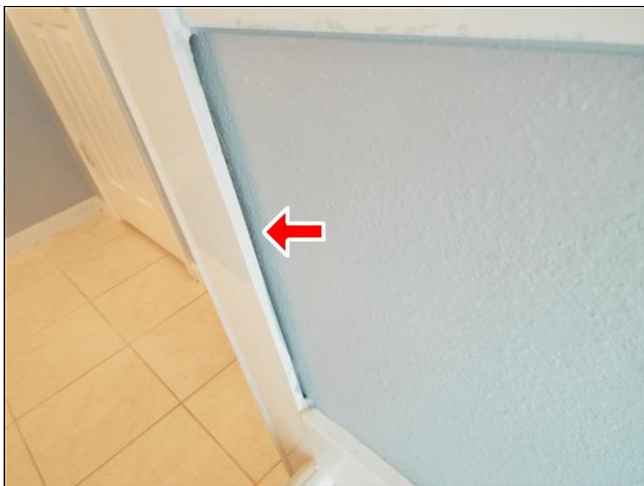
F. Item 38(Picture) The corner over bath tub is in need of sealing at opening.
