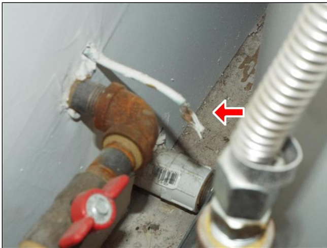
B. Item 5(Picture) Ground does not appear to be properly connected.
