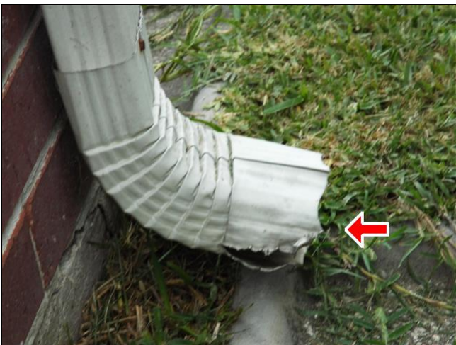
B. Item 1(Picture) Downspout end is damaged.
