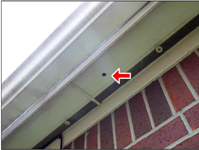
F. Item 7(Picture) Hole inside soffit board is in need of sealing.
