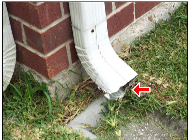
B. Item 2(Picture) Downspout end is damaged.
