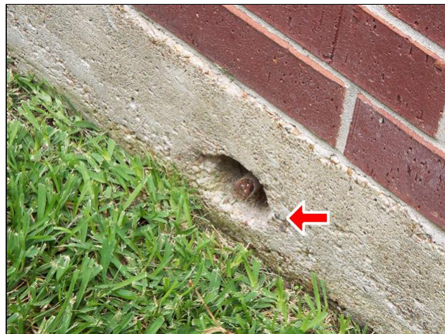
A. Item 4(Picture) Post tension holes along the foundation perimeter needs filling.
