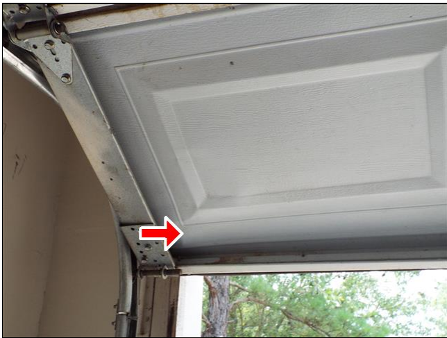
G. Item 3(Picture) The right bottom corner of garage is damaged.
