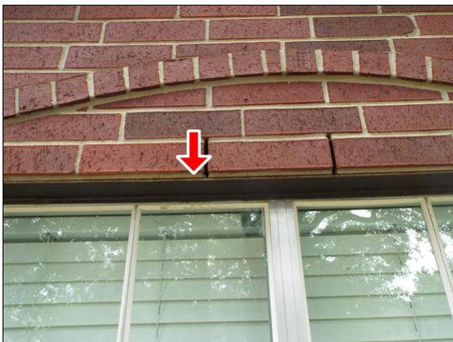
H. Item 3(Picture) Lintel is in need of sealing and painting
