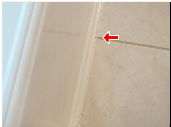
F. Item 39(Picture) The corner of floor tile and wall is in need of sealing.
