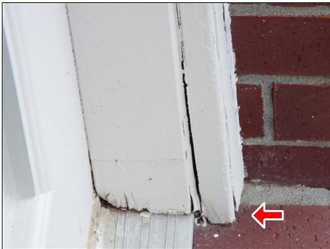
F. Item 25(Picture) Wood needs repair around rear door.
