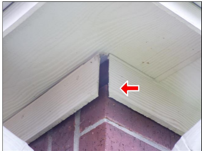
F. Item 10(Picture) Corners of brick fascia boards shows separation and seams are in need of sealing and painting. Repair is needed.
