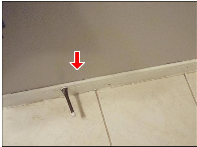
E. Item 2(Picture) Base board is in need of sealing in hall bathroom.
