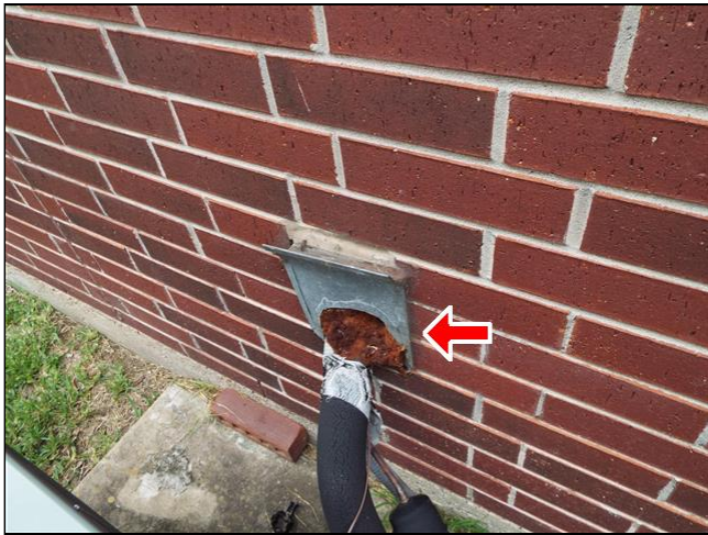
B. Item 1(Picture) Penetratyon needs filling.
