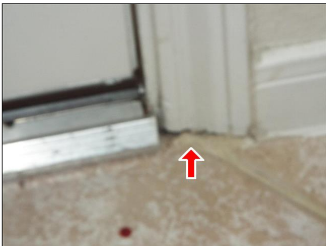
F. Item 42(Picture) Caulking is needed at the base of front door trim board.
