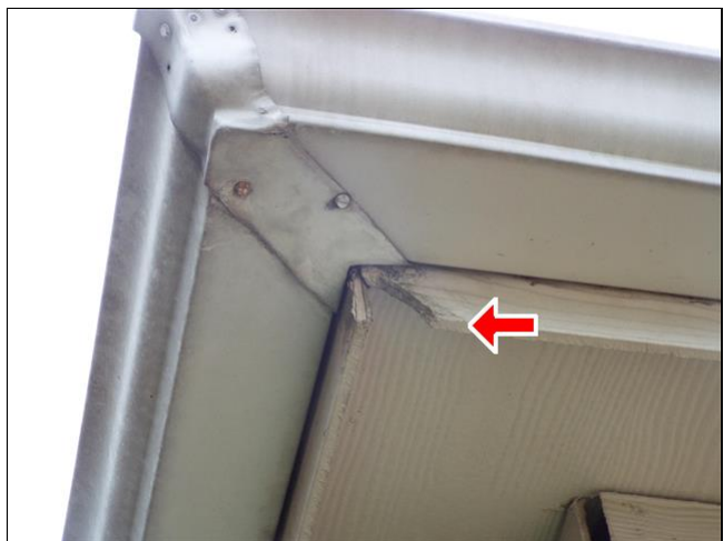
F. Item 6(Picture) Fascia board corner is damaged and is in need of repair.
