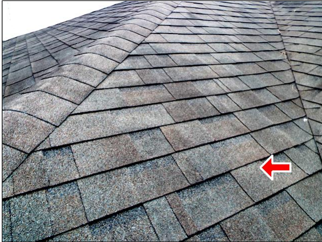
C. Item 1(Picture) Shingle edges appears to expose fibers.
