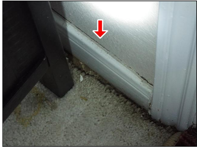
F. Item 35(Picture) Base board is in need of sealing and painting near rear door.
