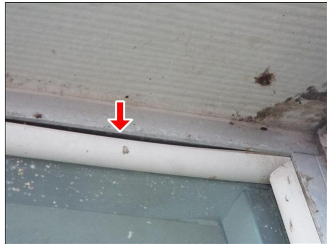
H. Item 2(Picture) Window seal needs to be repaired.
