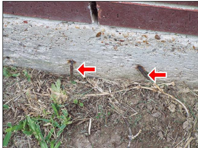
A. Item 2(Picture) Nails need to be cut along the foundation perimeter.
