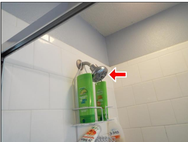
A. Item 3(Picture) Shower heads needs repair.
