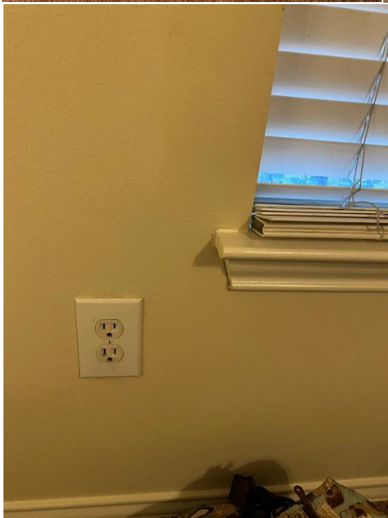
P20, 3: Outlet - Loose Cover Plate - Attic Fix: secured screw
