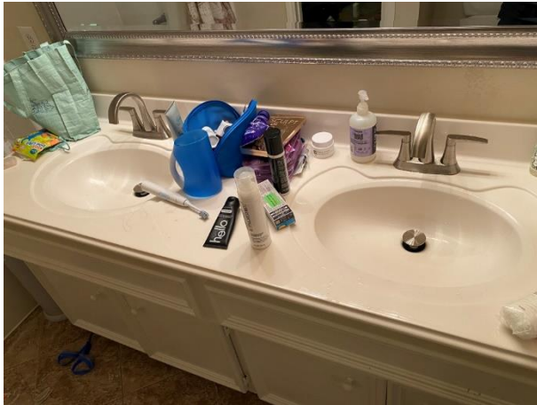
P28, 3: Sink - Slow Drainage (adjust drain stop)
