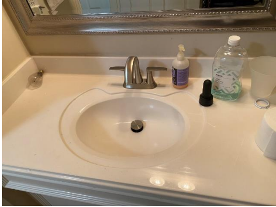
P28, 3: Sink - Slow Drainage (adjust drain stop)
