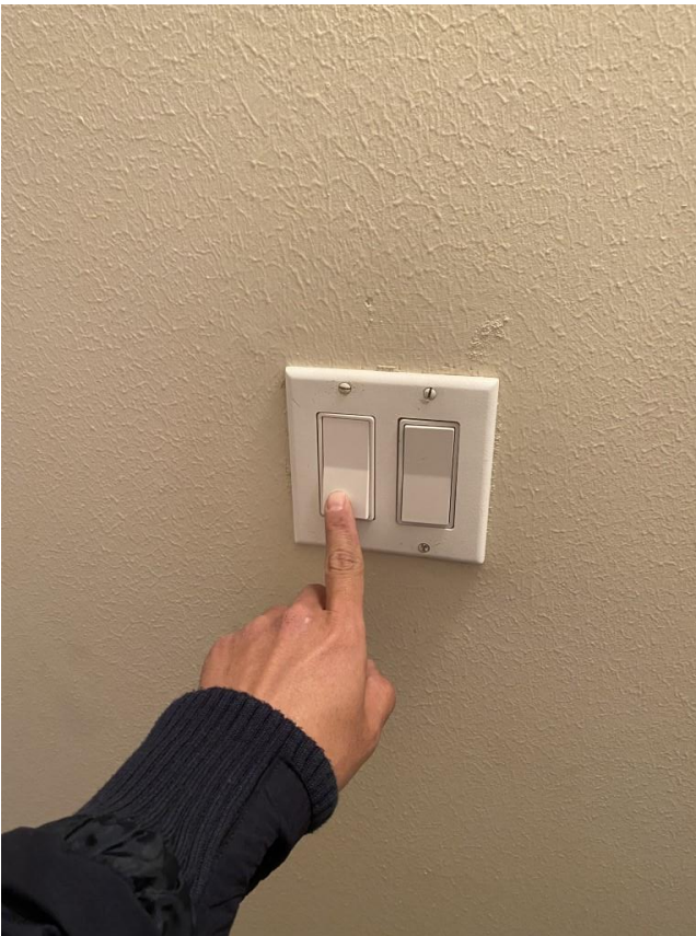
P21, 9: Switch - Not Functional Fix: replaced with larger flat switches
