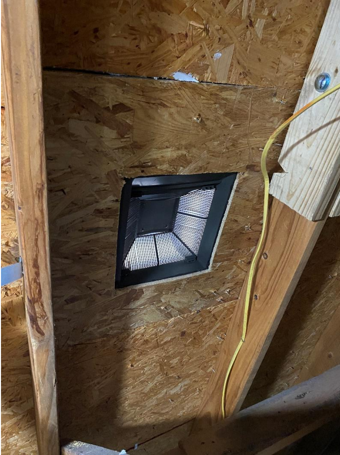
P8, 7: Loose Hardware At Attic Ladder Fix: Nuts were tightened
