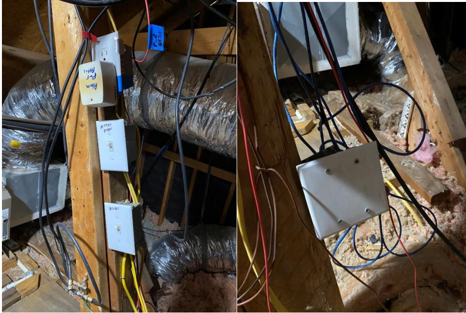
P20, 4: Smoke Detectors - Older Fix: replaced old smoker detectors
