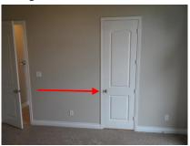
The master bathroom door does not latch properly. The door must be pushed fully closed to latch properly. Adjustments are needed at the striker plate.
