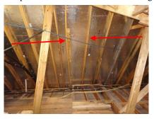
• The radiant barrier sheathing is damaged or has peeled away at the furnace vent roof penetration.
