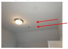
Possible missing, inadequate or improperly installed insulation was observed at the living room ceiling (and possibly wall) at the left front corner of the master bedroom. The colder wall section is an exterior wall and may be insulated.
