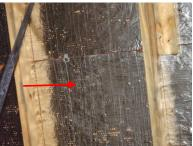
• Warped rafters were observed at the right side slope of the roof near the attic entrance.
