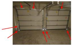
The weather seals are unfinished around the exterior of the overhead garage doors.
