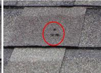
The right side roof slope is uneven or is buckling in several locations. Repairs should be undertaken as necessary.
