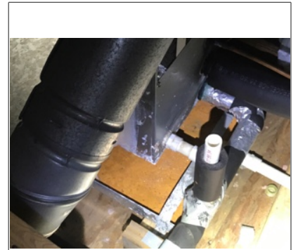
Clean rust in pan
