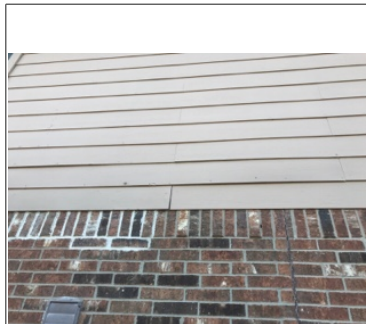
Siding needs repairs and seals at seams
