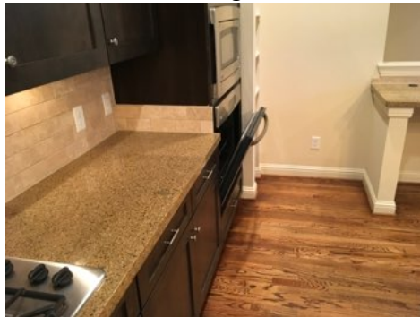
Not GFCI protected
