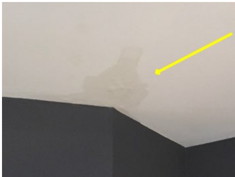
Evidence of moisture intrusion
