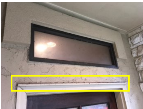
Wall sealed to flashing
