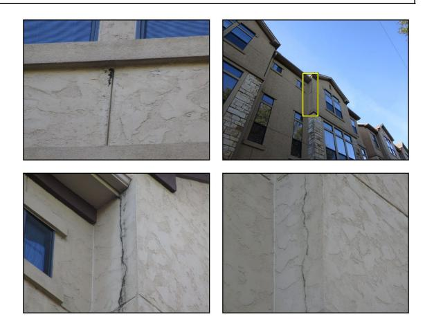
Inadequate space and/or missing weep screed at the base of the stucco. "Corrosion-resistant weep screed or plastic weep screed, with a minimum vertical attachment flange of 3½ inches shall be provided at or below the foundation plate line on exterior stud walls per the ASTM C 926. The weep screed shall be placed a minimum of 4 inches above the earth or 2 inches above paved areas and shall be of a type that will allow trapped water to drain to the exterior of the building." Per IRC R703.6.2.1.
