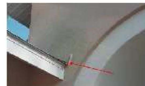
Fig 4: Proper repair kickout installation
