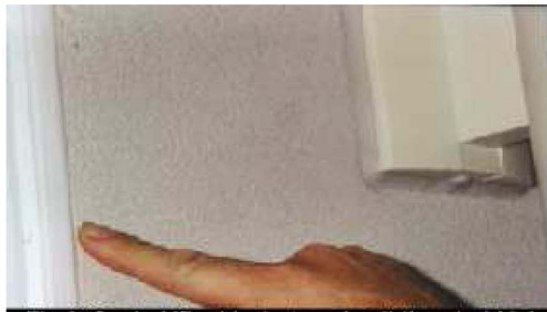
Fig. 3: Sealed 'flush' window detail (band-aid joint)
