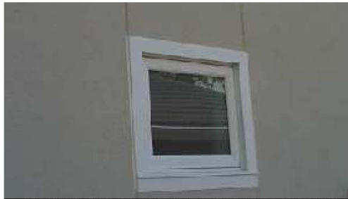
Figure 2: Typical outset window detail (sealed)
