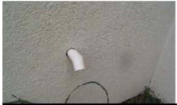
Fig. 1 Unsealed penetration
