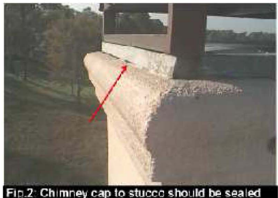
Fig.2: Chimney cap to stucco should be sealed
