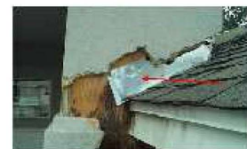
Figure 3: Failed flashing
