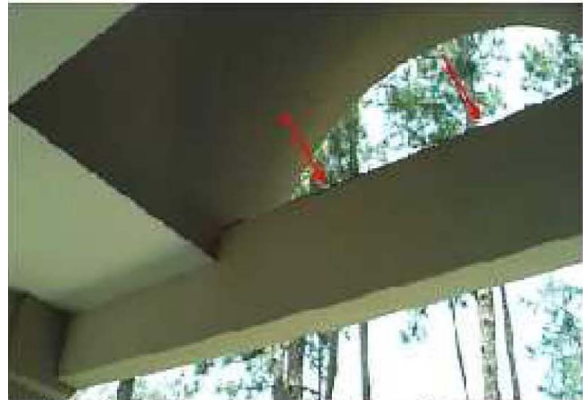
Fig. 2: Flat surfaces on top of beams
