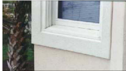
Figure 1: Typical inset window detail (sealed)
