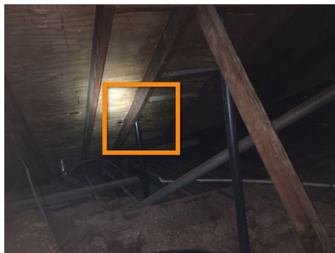
Sewer vent over the hallway bathroom
