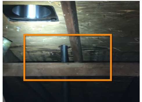
Sewer vent at the west side of the attic
