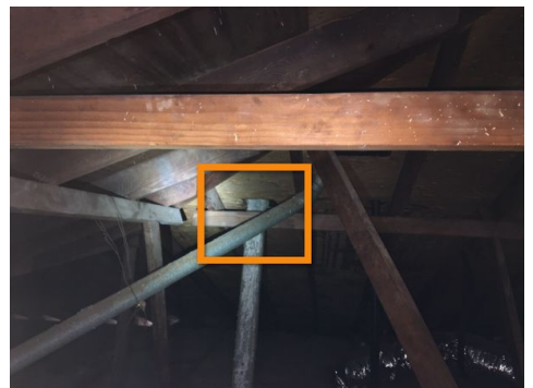
Vent at the west side of the attic
