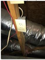
Issue: Receptacle obstructed in the garage. Recommend making fully accessible.
