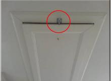
Issues: The door does not latch properly in the upstairs back left bedroom; recommend adjusting the strike plate for proper operation at minimum.
