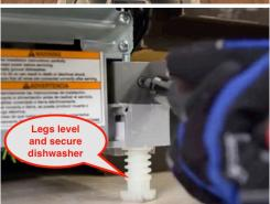
DEFICIENCY: The dishwasher is not secured at the bottom and moves when the dishwasher door is opened or closed. Adjusting the front legs will keep the dishwasher level and fully secure in the cabinet.
