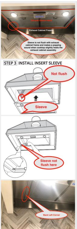
DEFICIENCY: The cooktop exhaust housing appears to be in a bind and the exhaust sleeve is not flush with the housing on the back left corner. The cooktop assembly makes a popping sound when it expands and contracts after being slightly heated by the gas cooktop burners below. (NOTE - The popping continues for several minutes after it starts).
