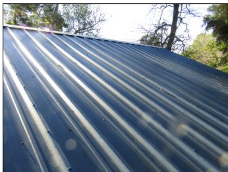
Roof appears to be in good condition.
