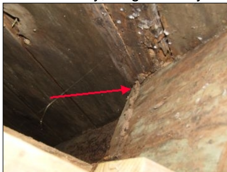
Mud tubes may indicate wood destroying insect activity.
