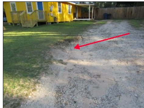
Needs pot hole filled and grading.
