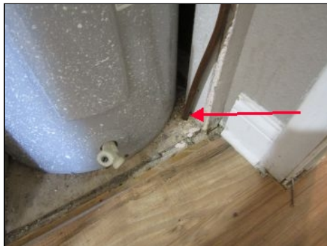
T & P drain pipe must have a visible discharge location.
