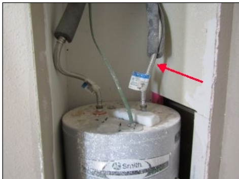
Water heaters are to have cold water shut off.
