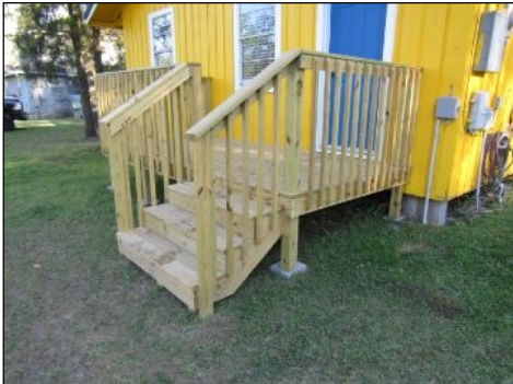
Front wood porch/deck appear in like new condition.
