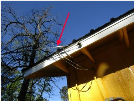
The service entry weather head does not have adequate clearance from the roof. Minimum distance of 3 ft. in all directions from edge of roof is required.
