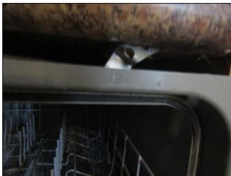
Not properly anchored to counter.
