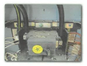
There is a white wire used as a hot conductor connected to the breaker for the A/C system. Normally the white wires are neutral. When used as a hot conductor, the white wires should be color coded.
