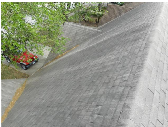
(2) General Photo of Roof Covering
