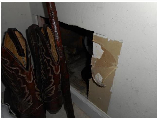
(5) Access panel covers are missing from master bathtub area.
