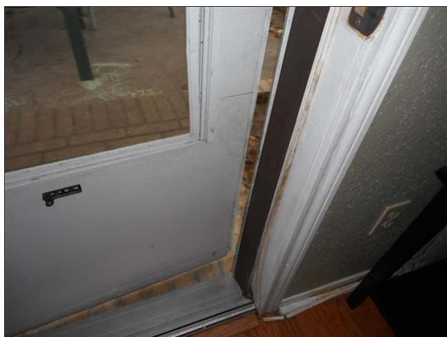
(2) Rear exterior storm door does not shut properly.
