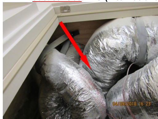
Sample of blanket insulation between ducts.
