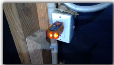
( In the car port storage area )
