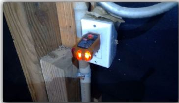
( In the car port storage area )
